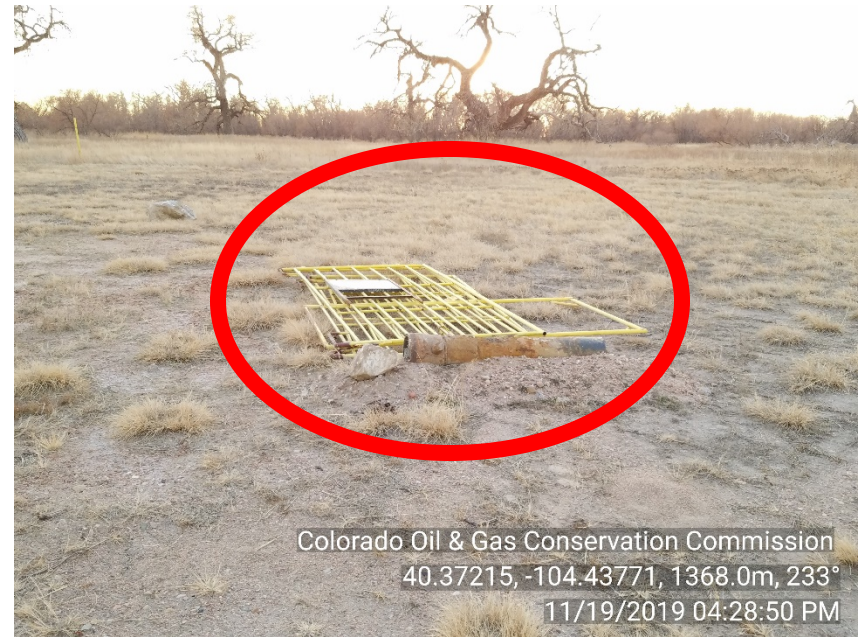
Photo #4 DOW 32-28 Wellsite Plugged & Abandoned | PA Junk Cut casing pipe, well fence
