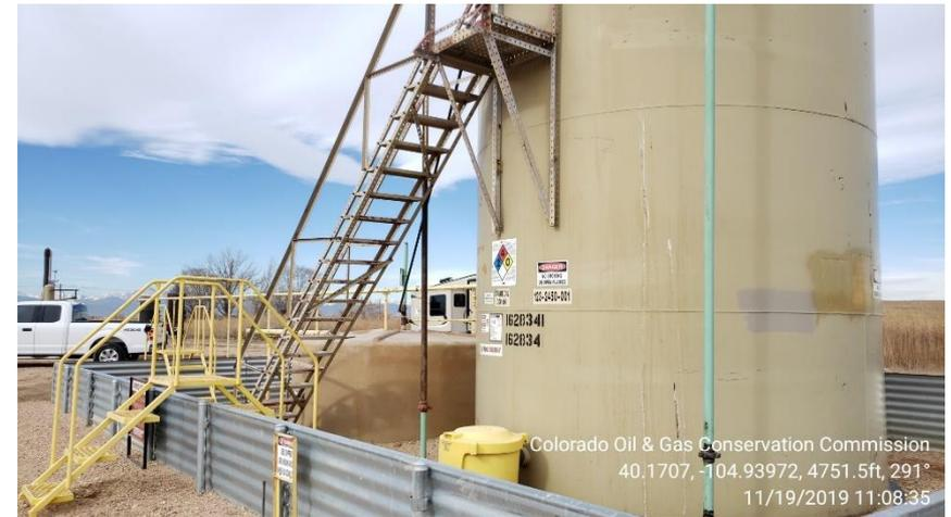
Photo 3 TB sign. No labels placards on produced water tank
