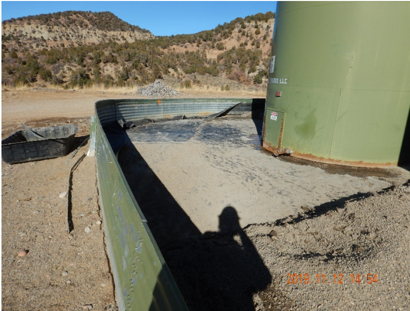
Photo #5 – View of partially-removed tank battery liner along northwest side of tank battery.
