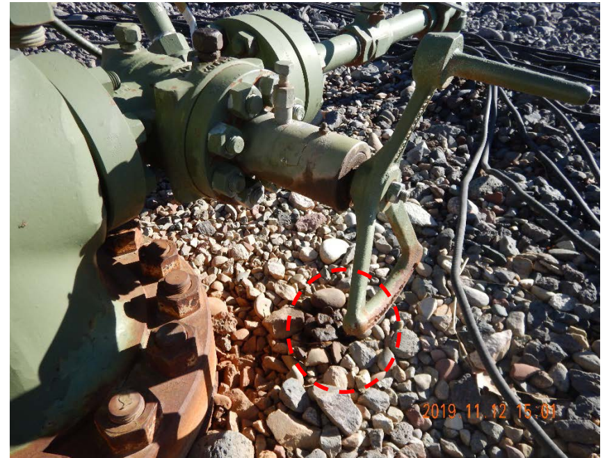
Photo #10 – Localized accumulation of oily waste (red circle) beneath valve attached to well #26-3C.
