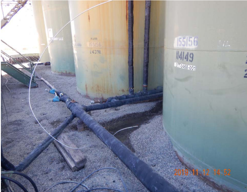
Photo #3 – View of unused process pipe in east side of tank battery secondary containment.
