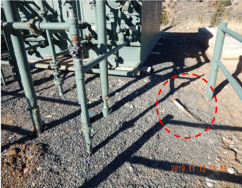
Photo #11 – Unused flowline daylighting southeast of separators (red circle).
