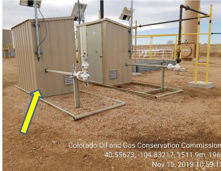
Photo 5: Gas meter disconnected.
