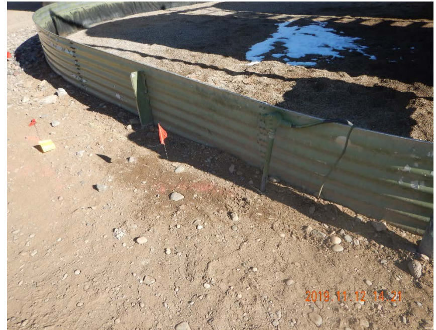
Photo #12 – Saturated soil observed west of central tank battery secondary containment.
