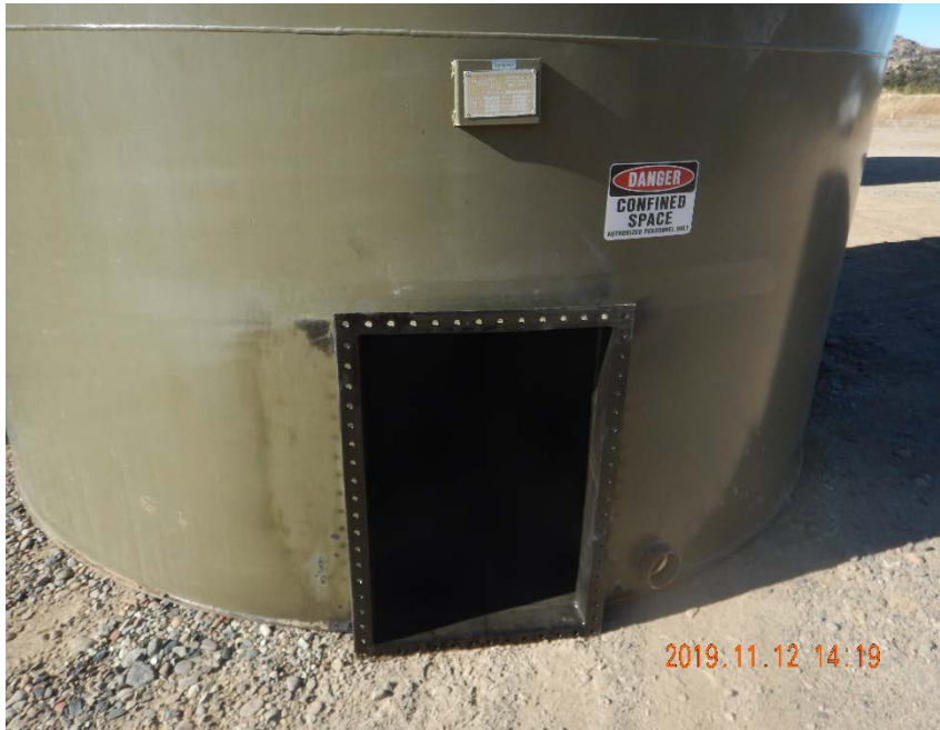
Photo #3 - Open access panel on unused steel AST (2).
