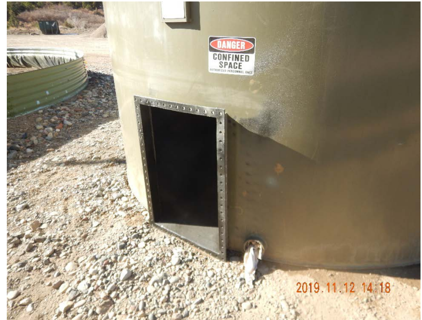
Photo #2 – Open access panel on unused steel AST (1).
