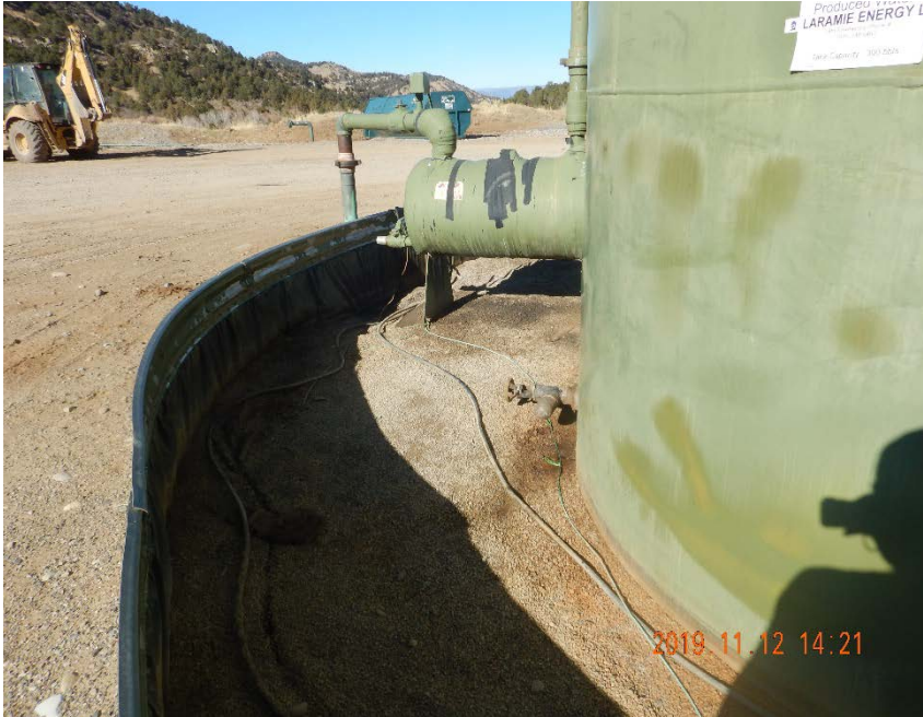
Photo #9 - Stained gravel inside of central tank battery containment (3).
