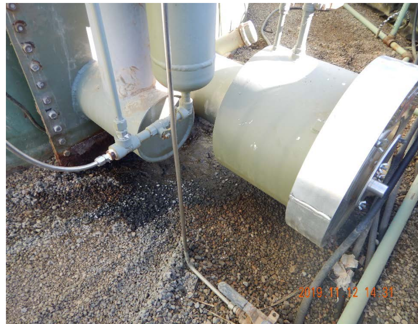
Photo #20 - Stained gravel inside of north tank battery containment (2).
