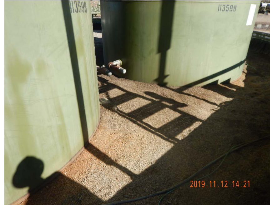
Photo #10 - Stained gravel inside of central tank battery containment (4).
