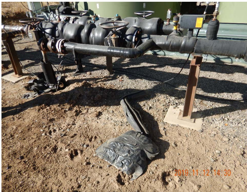
Photo #23 – Junk insulation located on south side of north tank battery.
