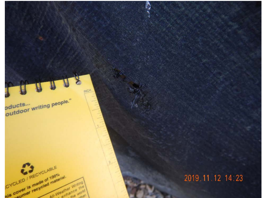
Photo #6 - Hole in liner at central tank battery, north side (2).
