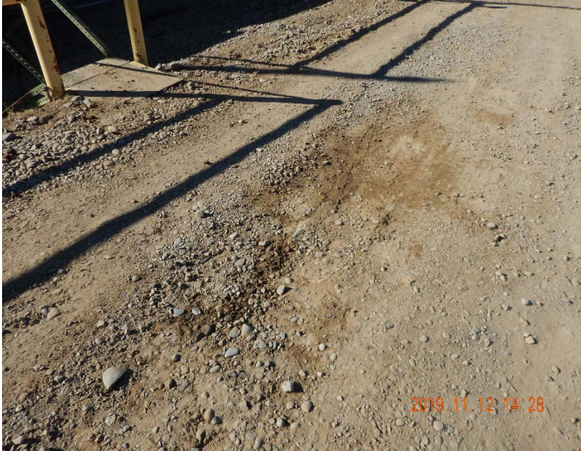
Photo #15 - Localized accumulations of oily waste along access road north of compressor station (2).
