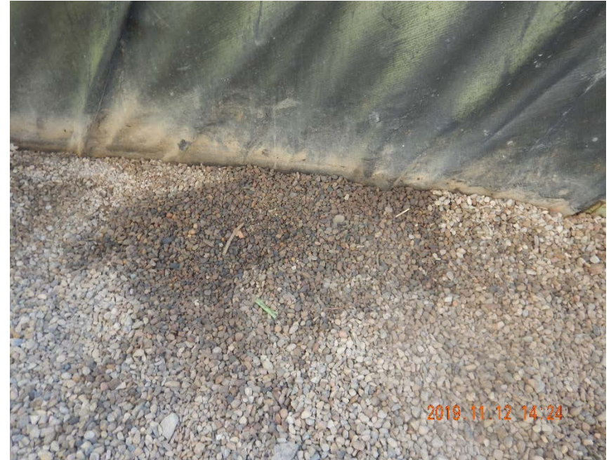
Photo #8 - Stained gravel inside of central tank battery containment (2).
