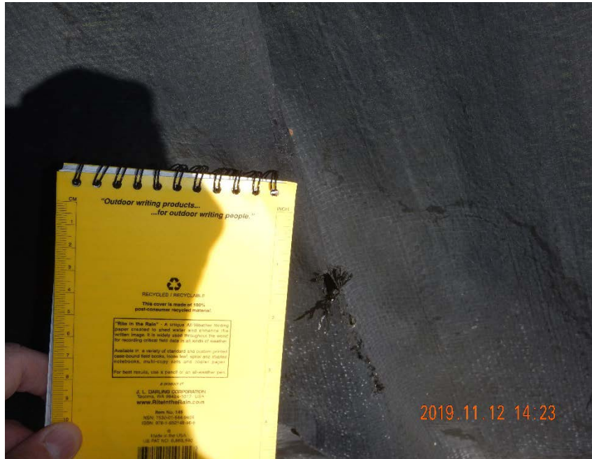
Photo #5 – Hole in liner at central tank battery, north side (1).
