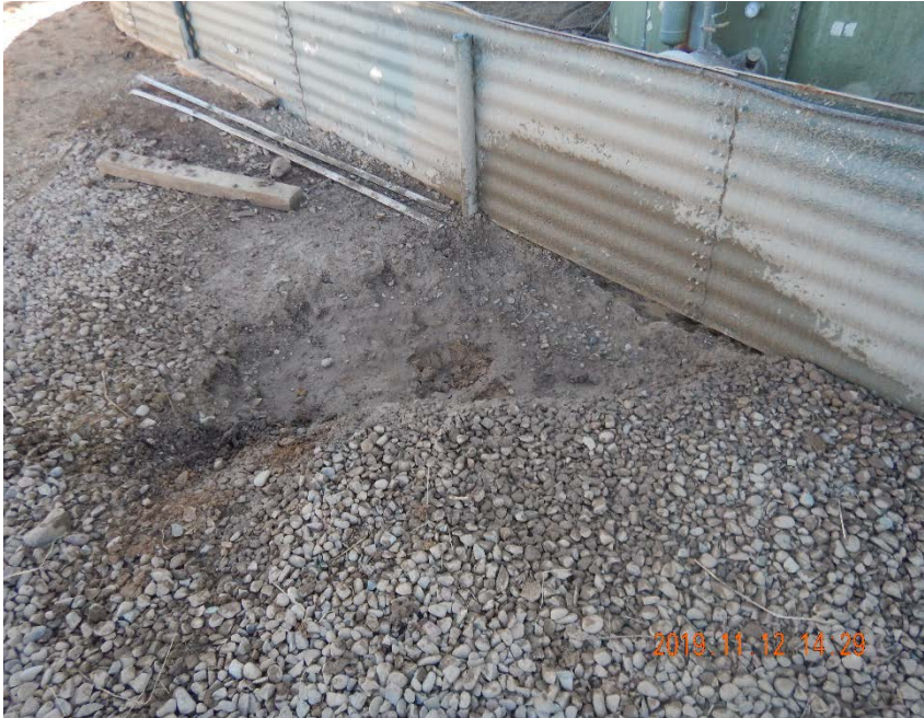
Photo #17 – Depression beneath metal containment ring on east side of north tank battery.
