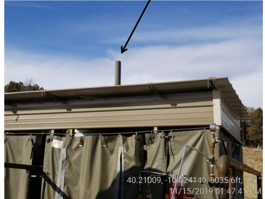
Photo 7. Stack with bird protection.
