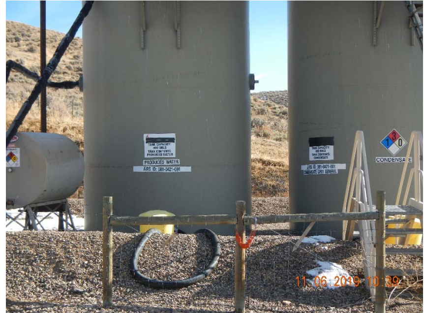
Photo 2. No NFPA diamond on produced water tank.
