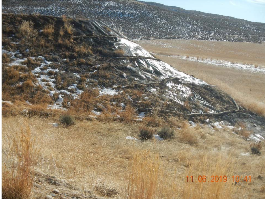
Photo 5. New wattles and netting on fill slope.
