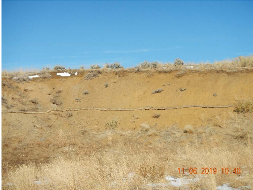
Photo 3. New wattles on cut slope.
