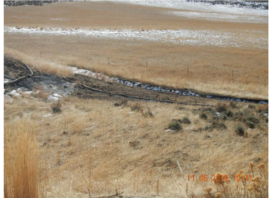
Photo 6. New wattles along ditch, no evidence of sediment migration.
