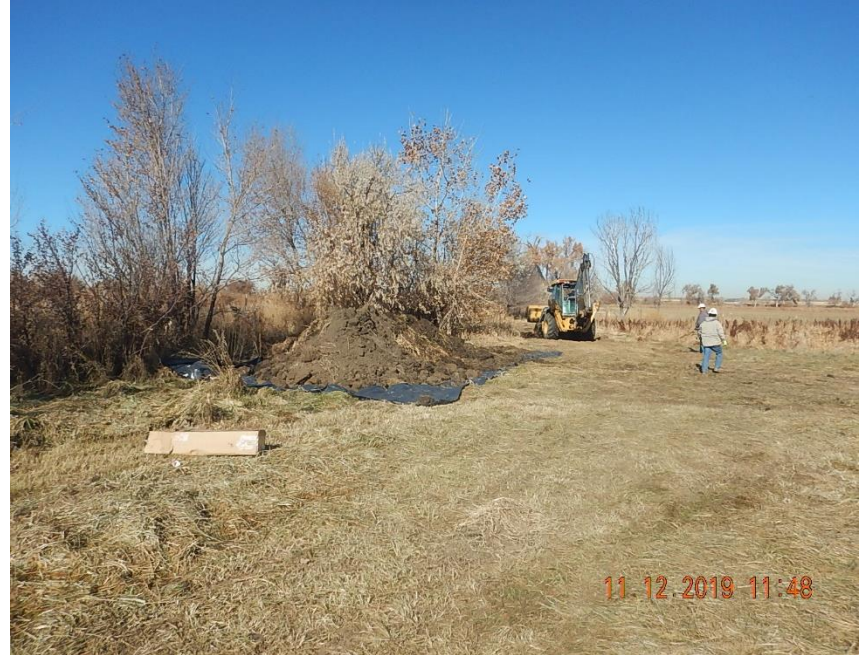
Spill response work in progress; impacted soils being removed.
