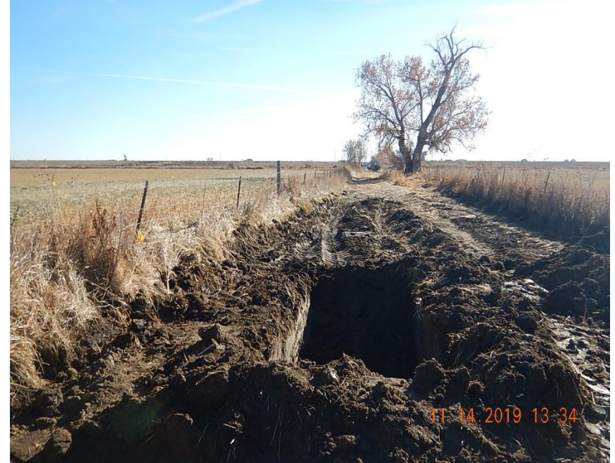
Bell hole excavation at release point; looking south toward second bellhole.
