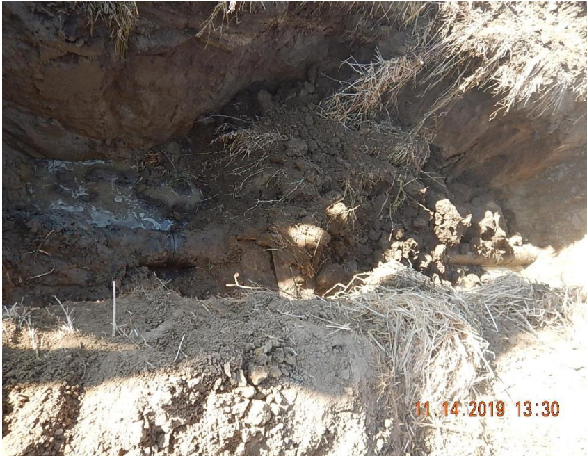
Close up view of 10" Facility #8 consolidation pipeline cut for repairs; exposed in south bellhole.
