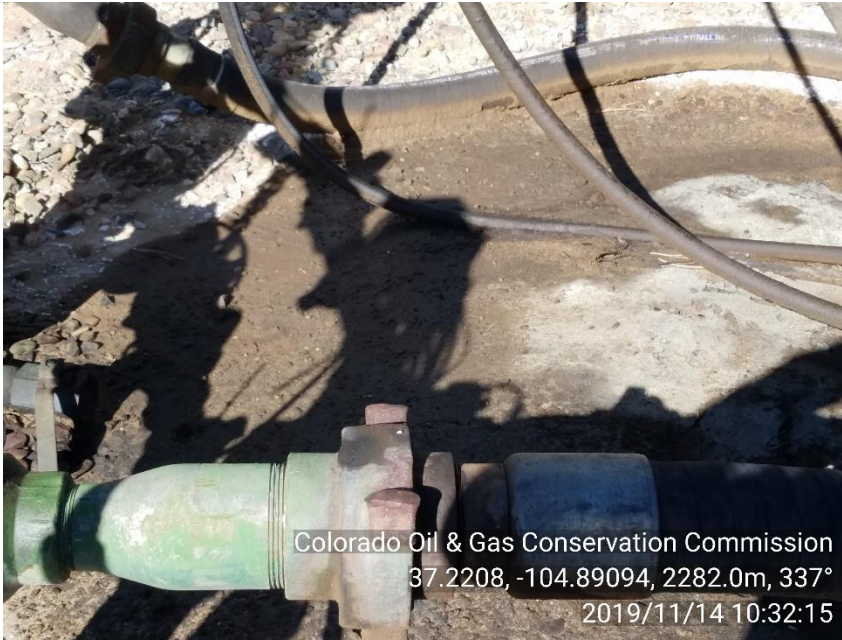
PHOTO 3: AREA OF IMPACTED SOIL NEAR WELLHEAD APPEARS TO BE OIL STAINED. Remove and dispose impacted material in approved manner, service and maintain equipment and self inspect to prevent recurrence of conditions per 1002.f(2) and 907. CA DATE 12-14-19
