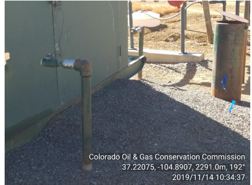
PHOTO 4: TWO UNUSED RISERS NEAR METER HOUSE. REMOVE UNUSED RISERS IN ACCORDANCE WITH RULE 603.f. AND NTO. CA DATE 2-14-20.
