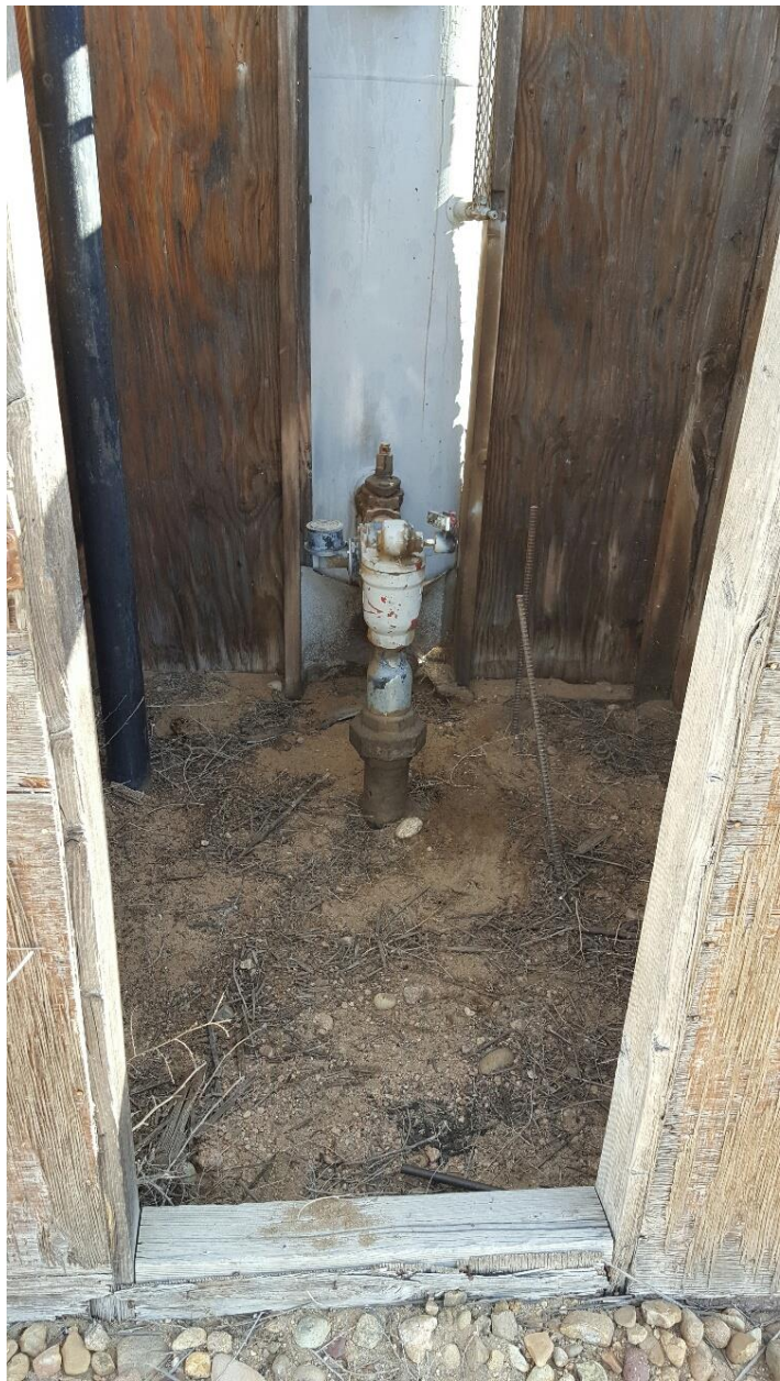
Figure #2 Risers have been bull plugged and labelled.
