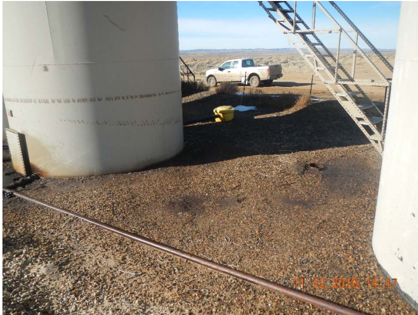
Photo 7. Free fluid and saturated soil in tank battery berm.
