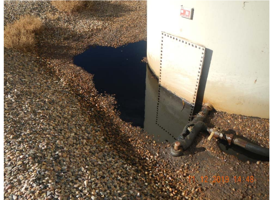
Photo 10. Free fluid and saturated soil in tank battery berm.
