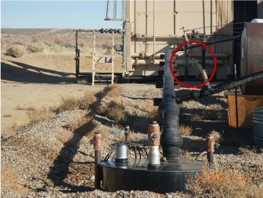
Photo 3. Ongoing vapor release with stained gravel below ball valve.
