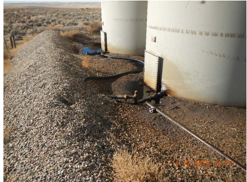
Photo 8. Free fluid and saturated soil in tank battery berm.
