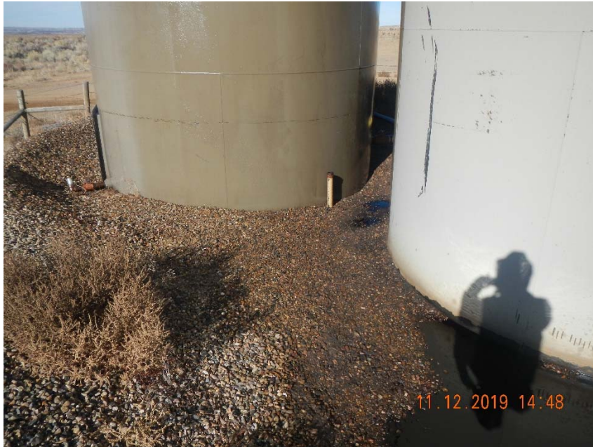
Photo 11. Free fluid and saturated soil in tank battery berm.
