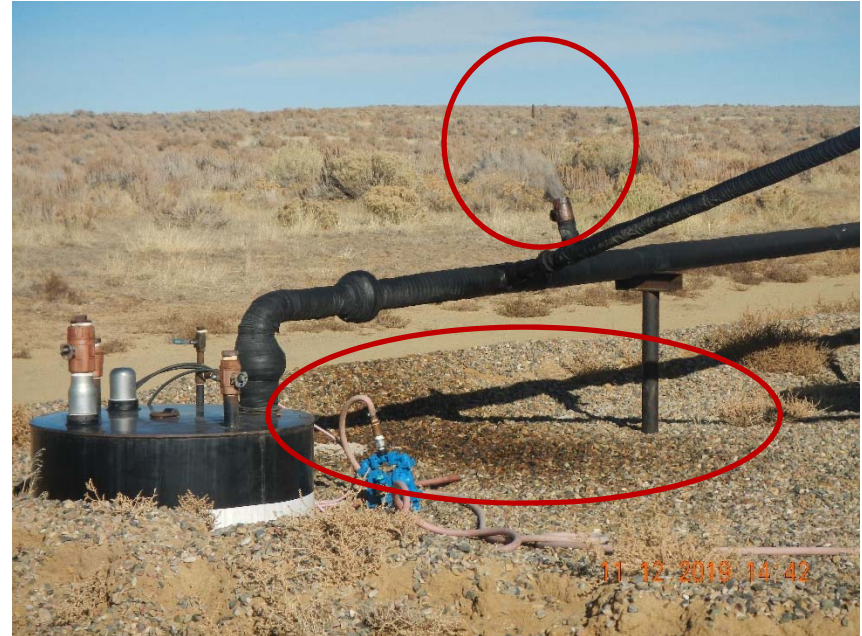
Photo 4. Opposite angle but still upwind of ongoing release from ball valve.
