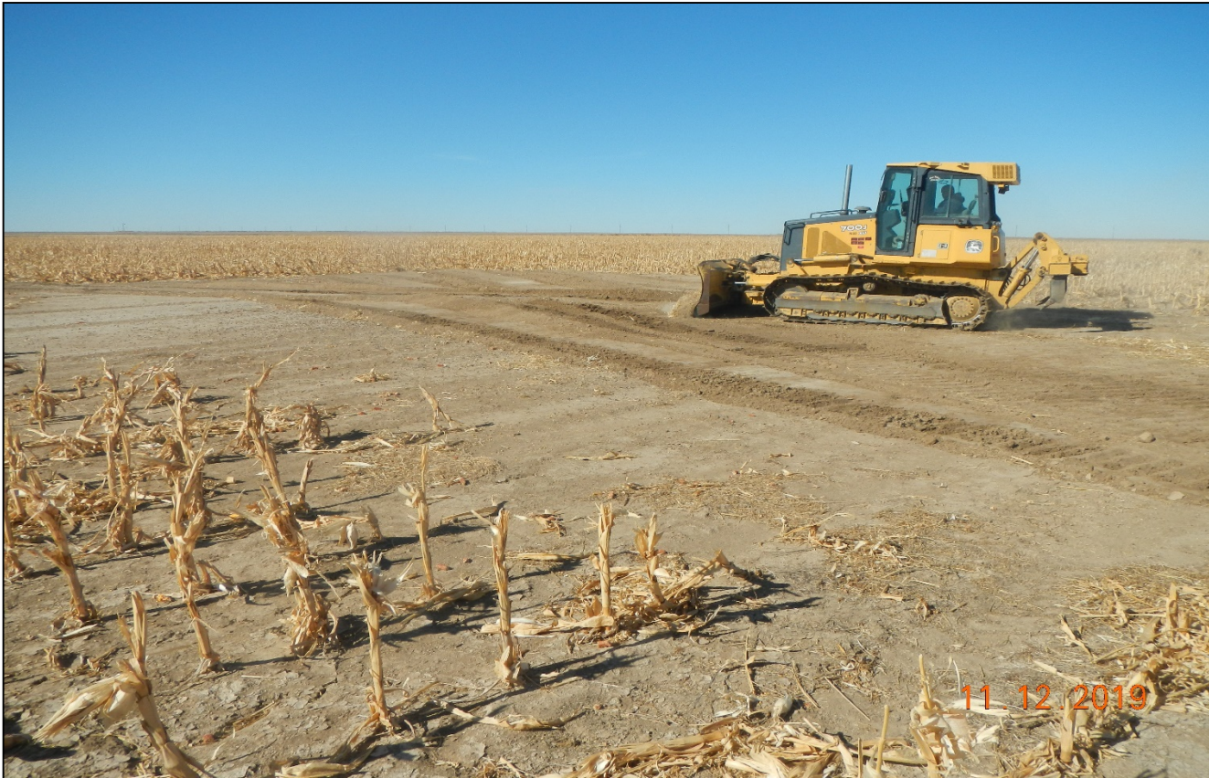
Photo 1. The location was leveled with the dozer.
