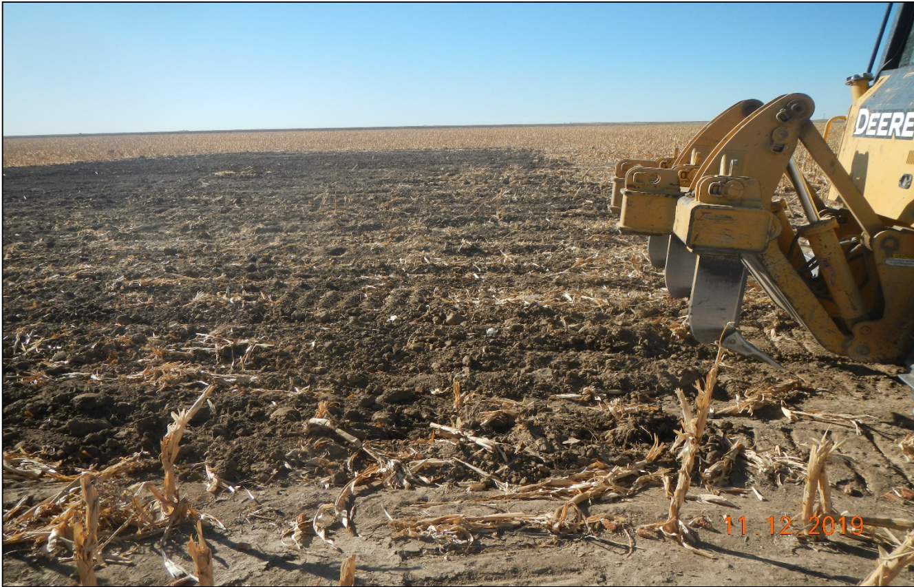
Photo 6. Facing west showing the area that was decompacted and the dozer ripper used for decompaction.
