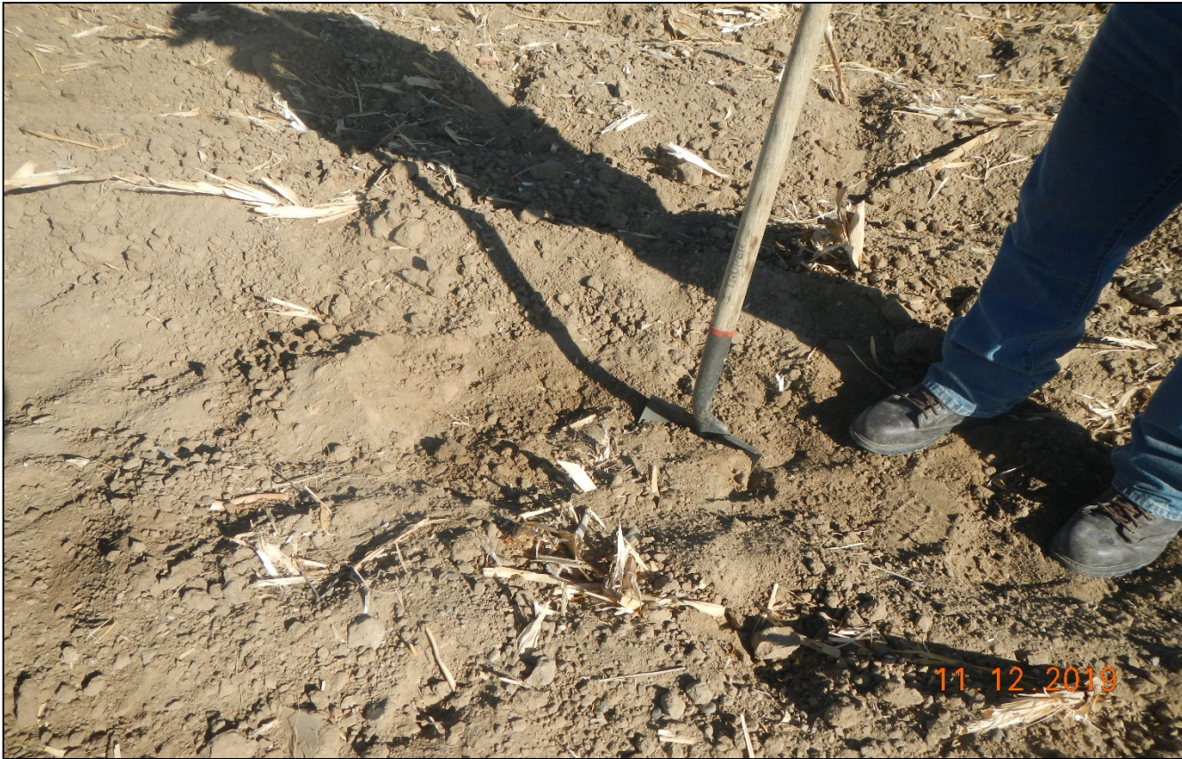
Photo 4. Soil was properly decompacted to 18 inches.
