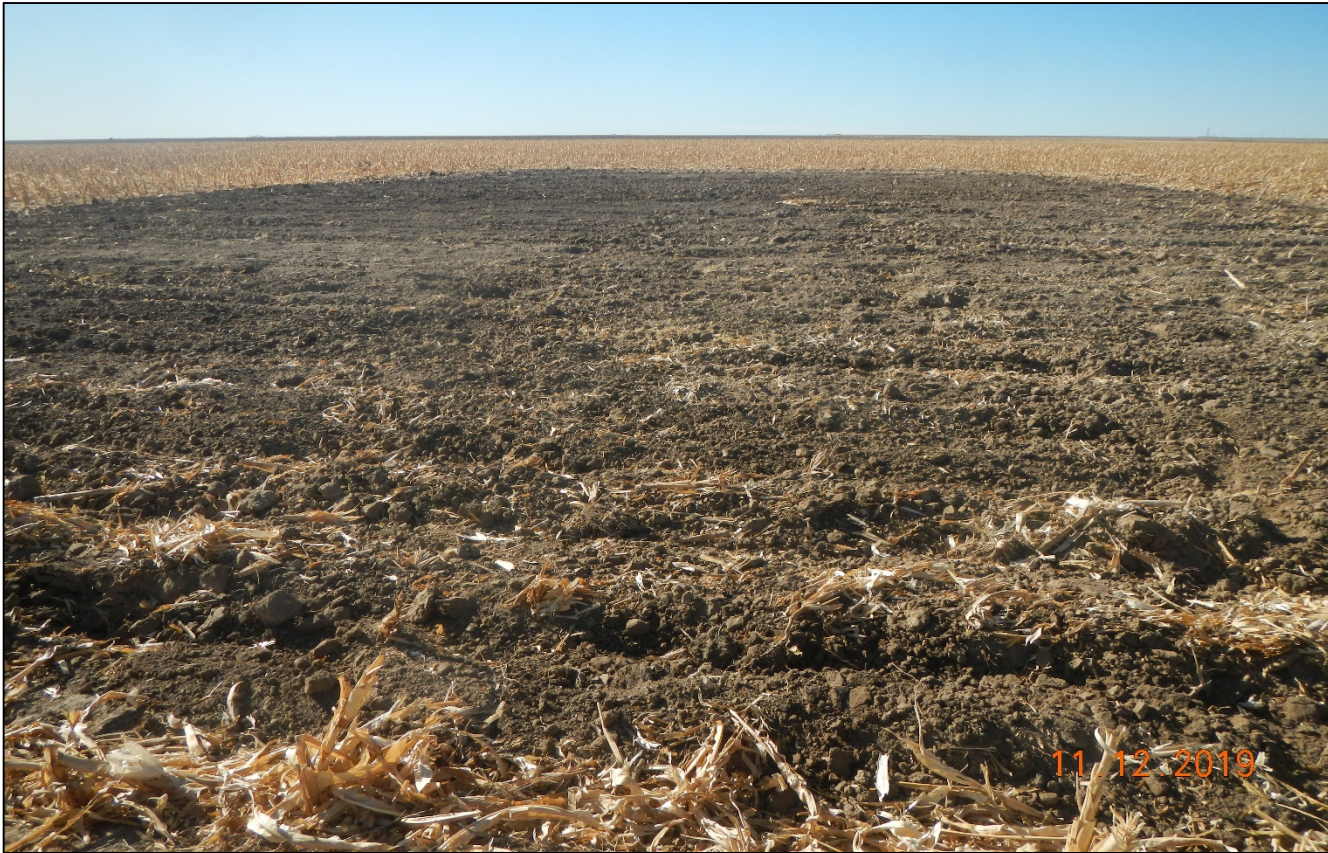
Photo 5. Facing west toward the location. The soils were cross ripped to 18 inches.
