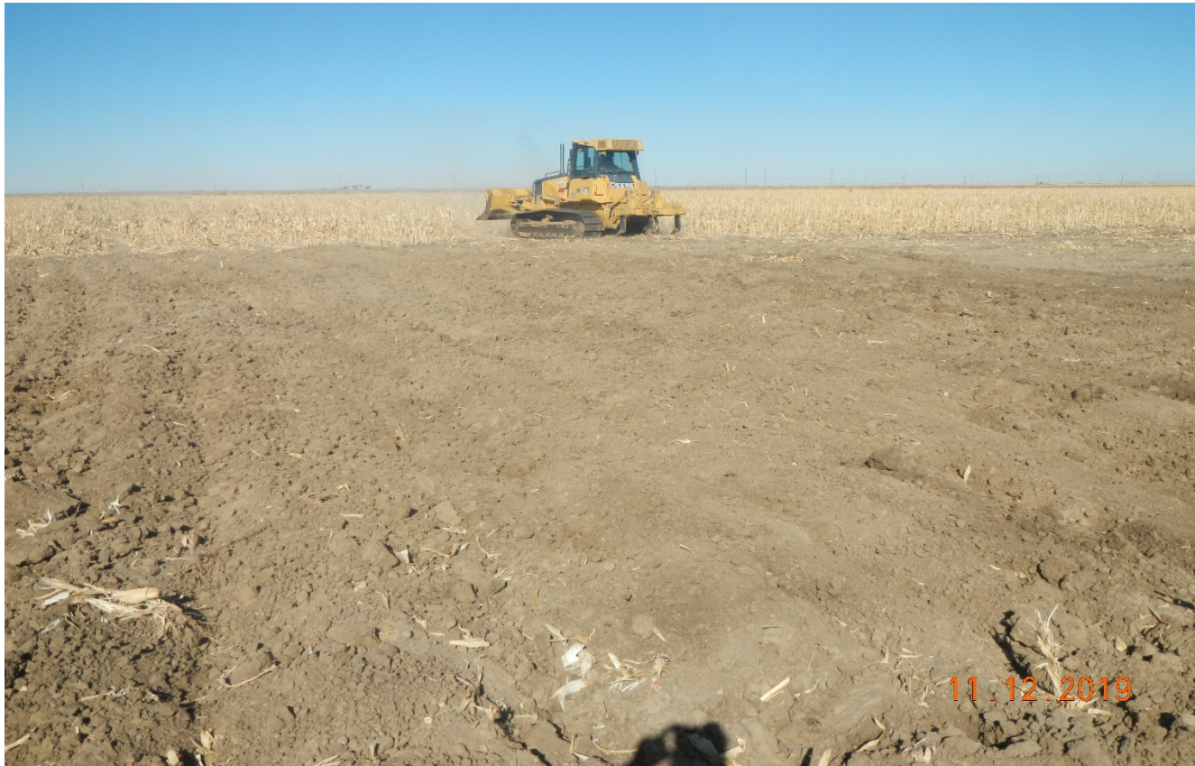
Photo 3. Cross ripping was performed from south to north.
