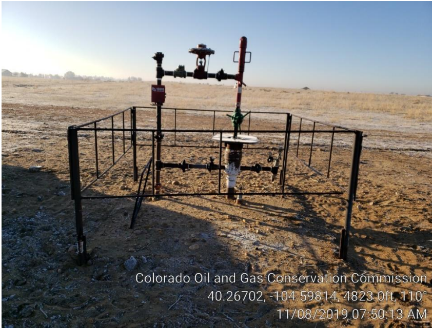
Photo #3 Wellhead & Missing sign. On 11/8/19
