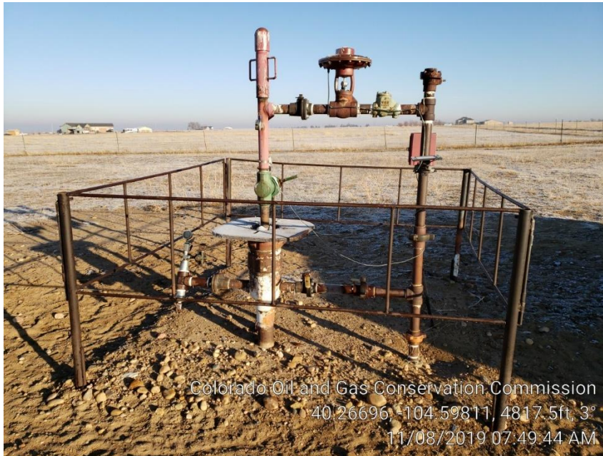
Photo #3 Wellhead & Missing sign. On 11/8/19
