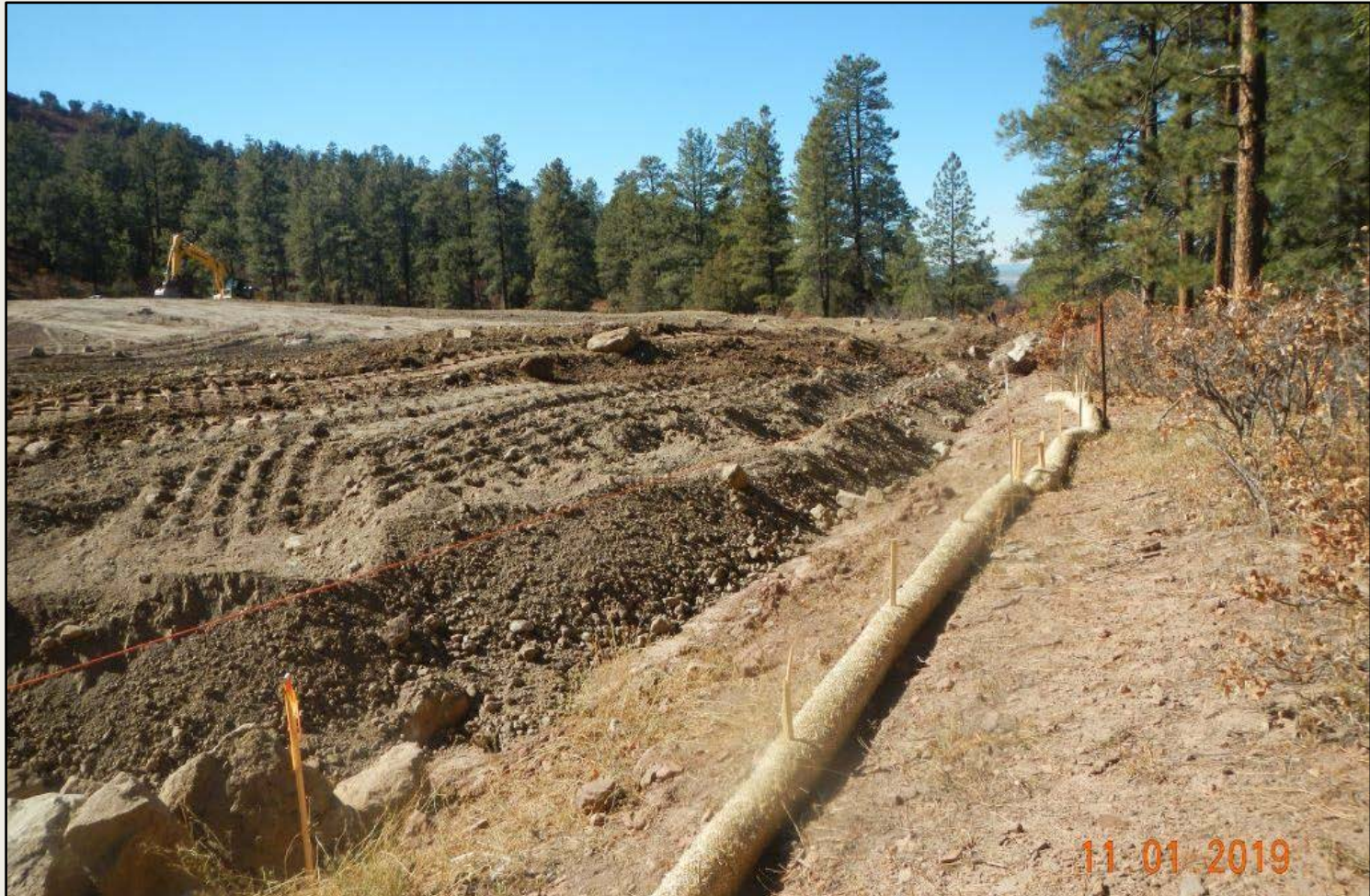
Photo 5. View of the northern project area from the northern corner facing westward. Wattles and trenching are in place.
