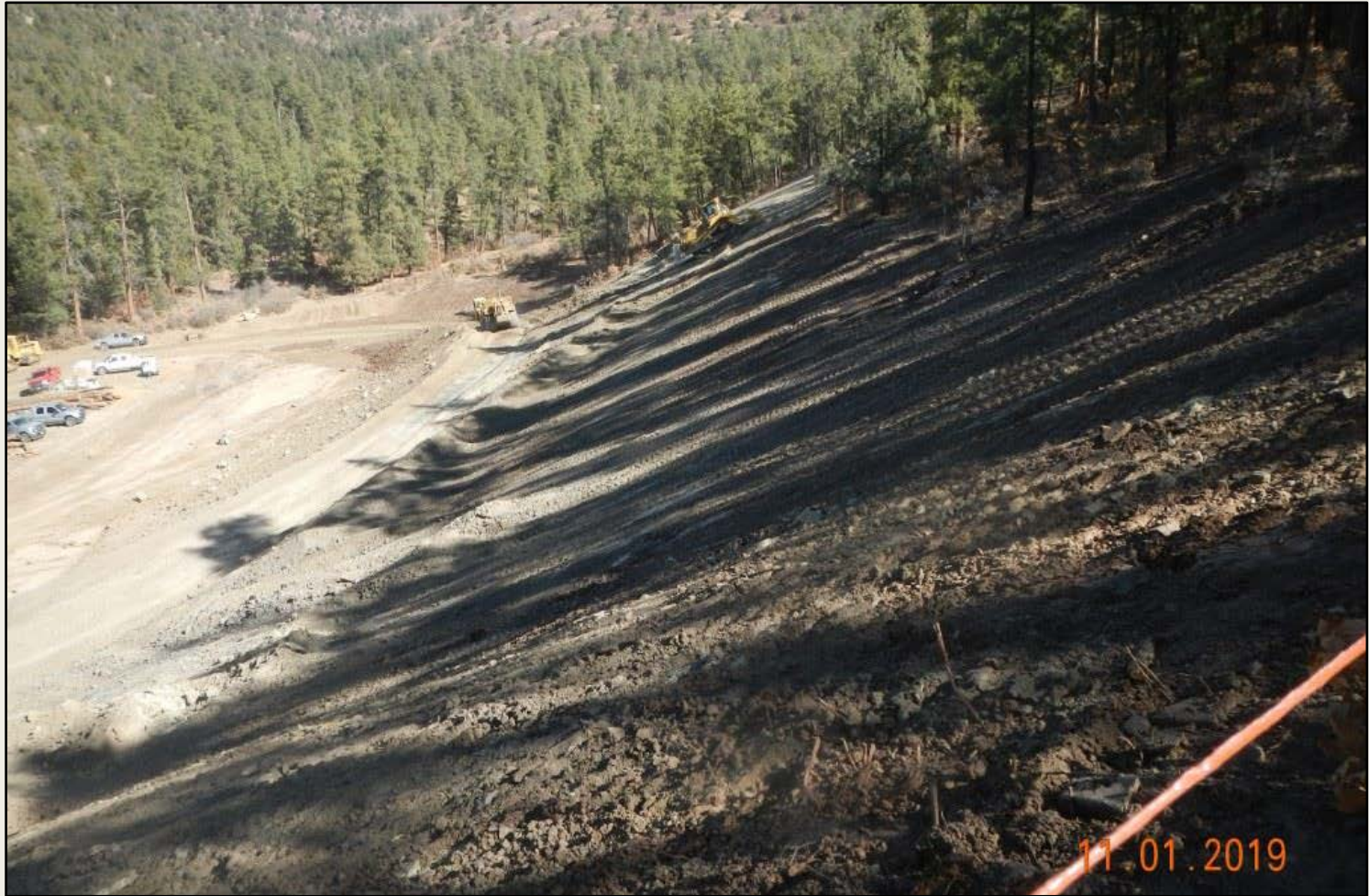
Photo 2. View of the southeastern cut-slope from the southern corner facing northward. Long-term stabilization measures will be needed to stabilize steep cut-slopes.
