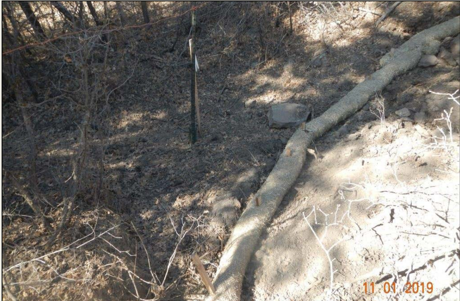
Photo 4. View facing downstream of Photo 3, within the southwestern project area, showing wattle/trench beneath topsoil and debris pile. These stormwater controls are not sufficient to contain volume of material upslope from here during a significant precipitation event. This area drains to an ephemeral drainage that flows toward Salt Creek.
