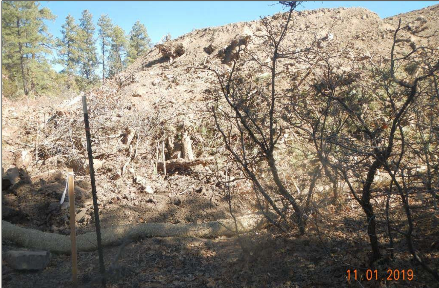
Photo 3. View of topsoil pile within the southwestern project area. Topsoil was in process of being moved to the northwestern project area, per communication with onsite construction staff. Stormwater controls in this portion of the project area are not sufficient to prevent downstream movement of sediment from soil and debris piles.
