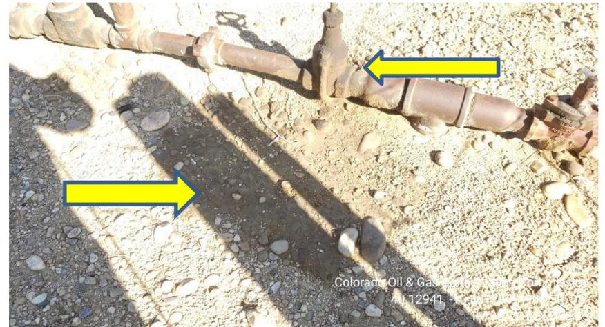
Photo 4 Stained soil by flow line valve on WH, Possible leak on valve
