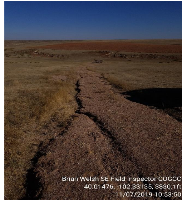
4. Erosion on access looking at location
