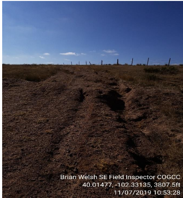
3. Erosion at BMPs that are washed out
