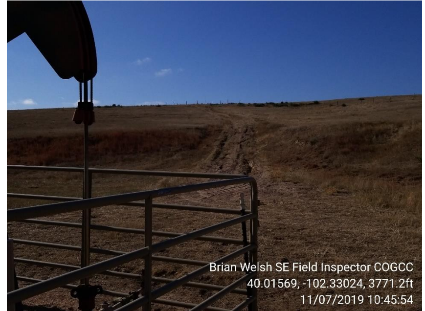
2. Access erosion near location
