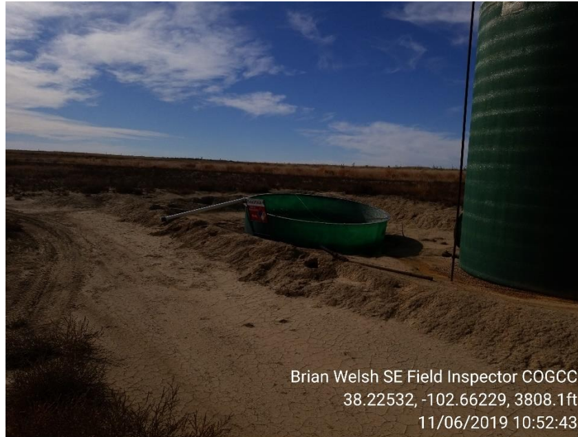
Erosion around leaning water tank
