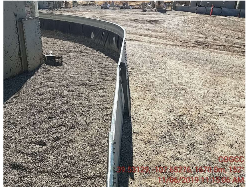
Damaged containment
