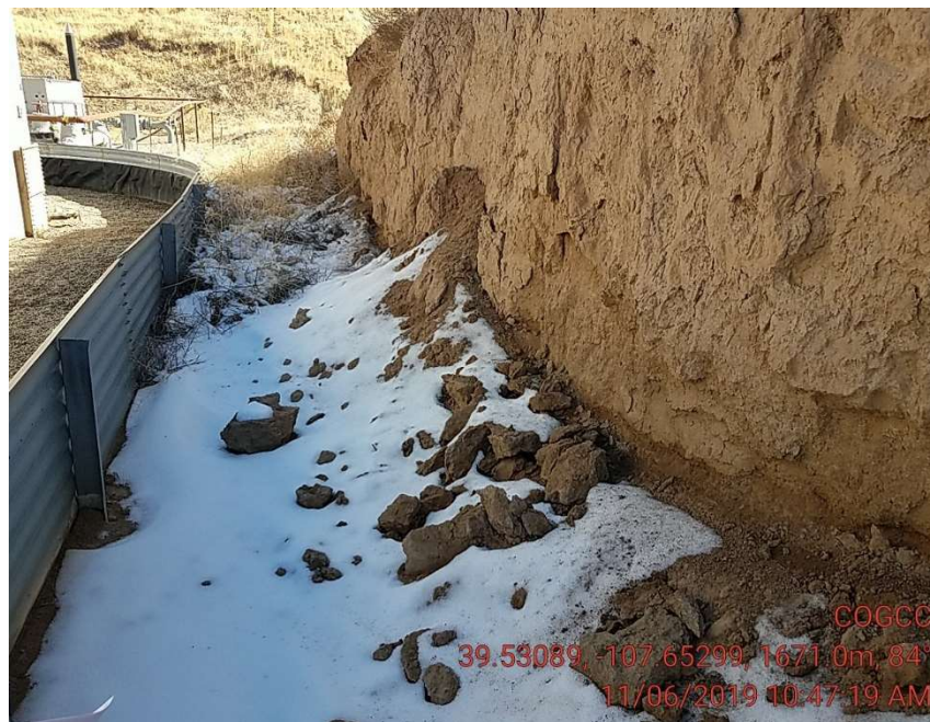
Needs slope stabilization (south side of pad)
