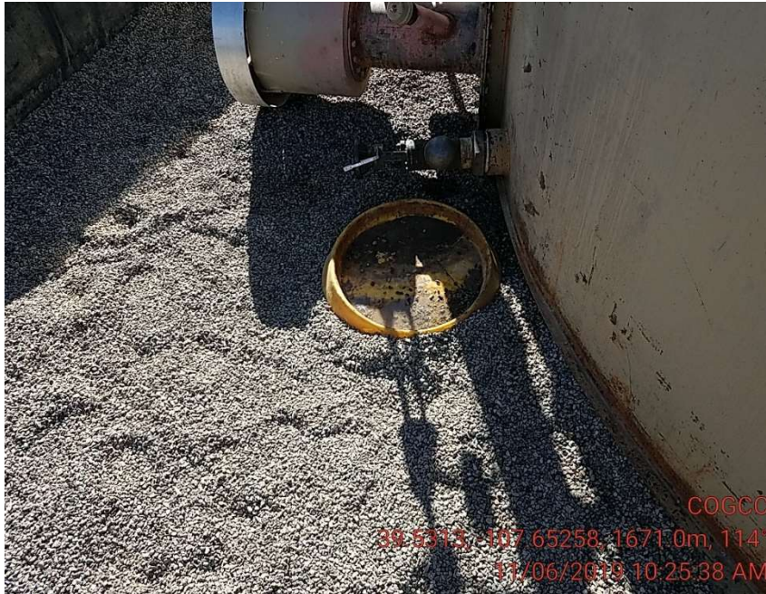
Fluid in drip pan next to lit burner
