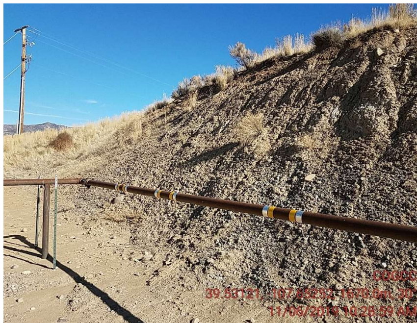
Needs slope stabilization (west side of pad)
