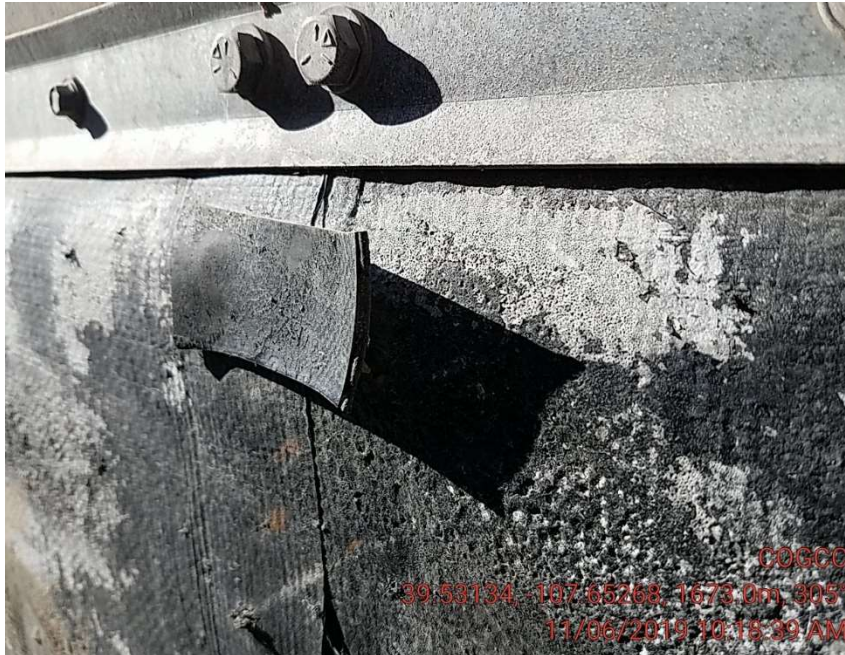
Liner patch not holding
