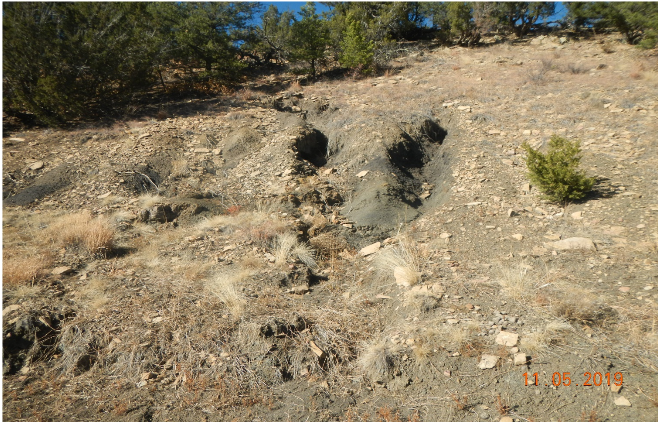
Photo 2. There is an area of erosion along the cut slope of the access road at Lat/Long:37.14248,-104.81373.
