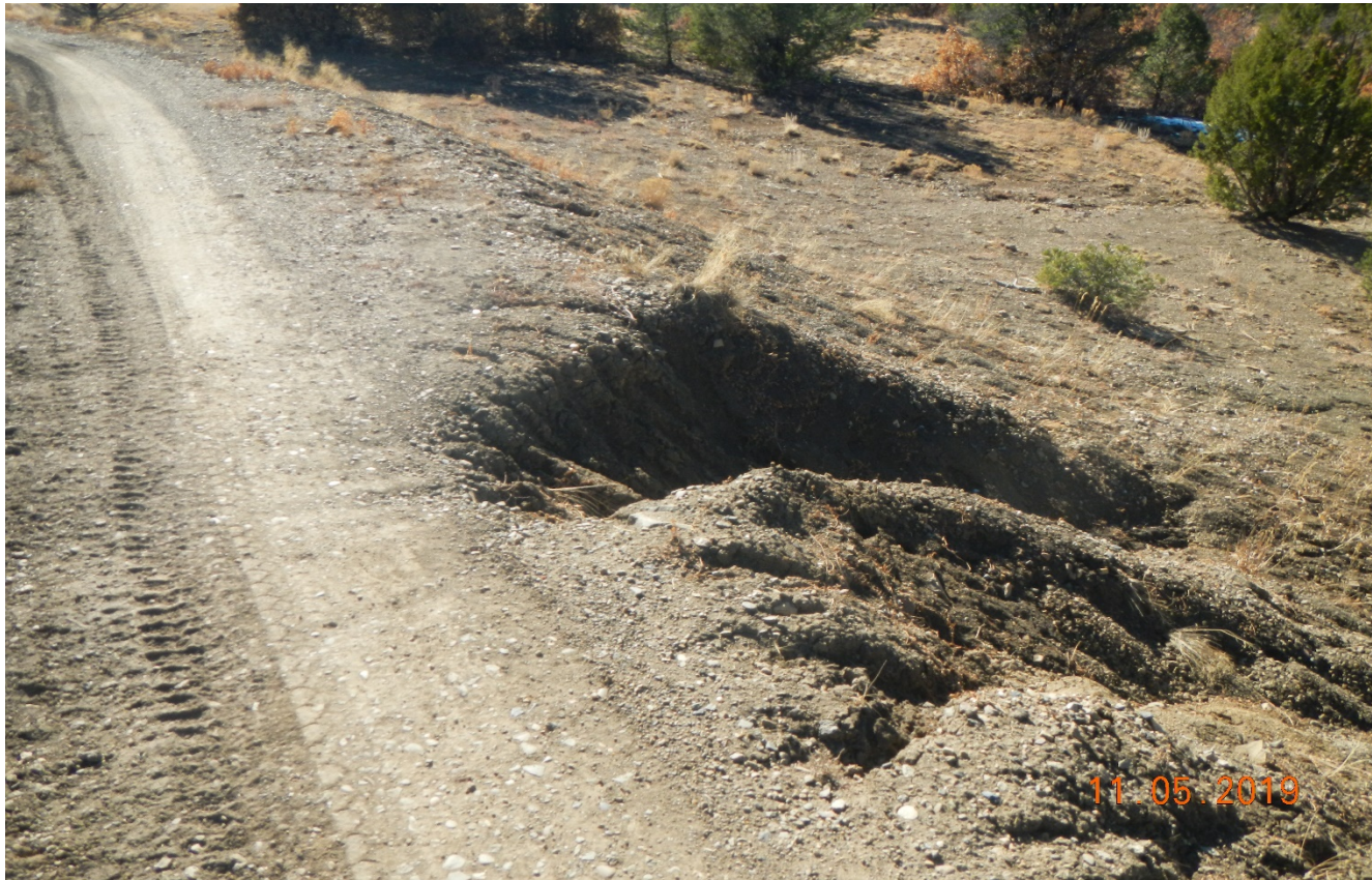
Photo 1. There is an area of erosion along the main road at Lat/Long:37.14023,-104.81186.
