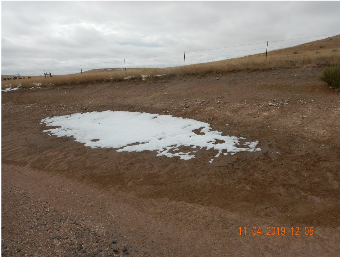
Photo 5. Photo taken from the western well pad, facing West. Operator claims that the western cut slope was properly stabilized. This photo illustrates that the cut slope has not been properly stabilized, as it remains in the same condition. There is no indication that a BMP has been installed or implemented.
