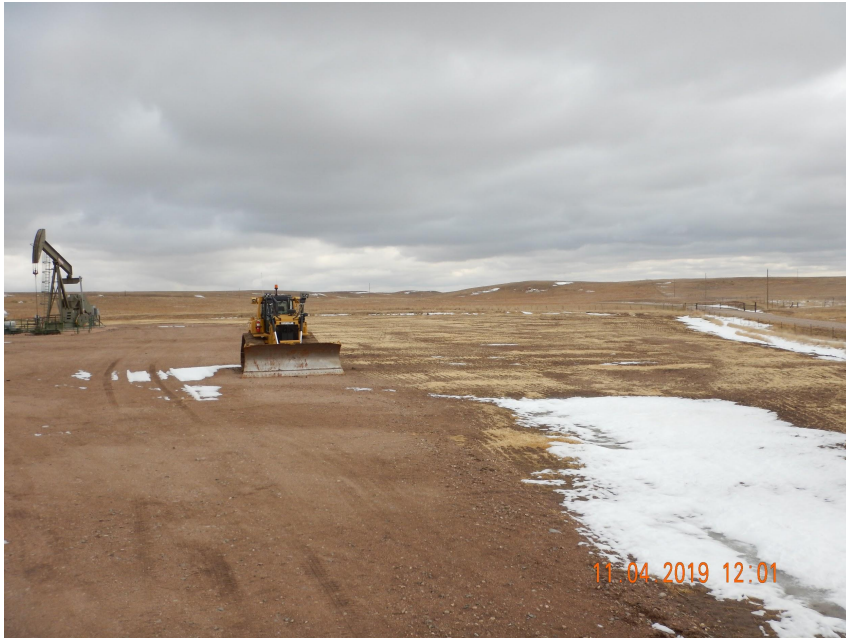
Photo 1. Photo taken from the entrance of location, facing East. Photo illustrates Operator has performed interim reclamation to reduce areas only needed for production operations per Rule 1003. Note: Appears straw mulch was crimped as an erosion control but has already blown off location which will not ensure the seeded soil is stabilized. COGCC staff would recommend re-installing erosion controls and using long-fiber weed-free mulch.
