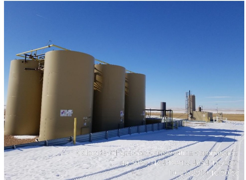
Photo 2 – Tank Battery
