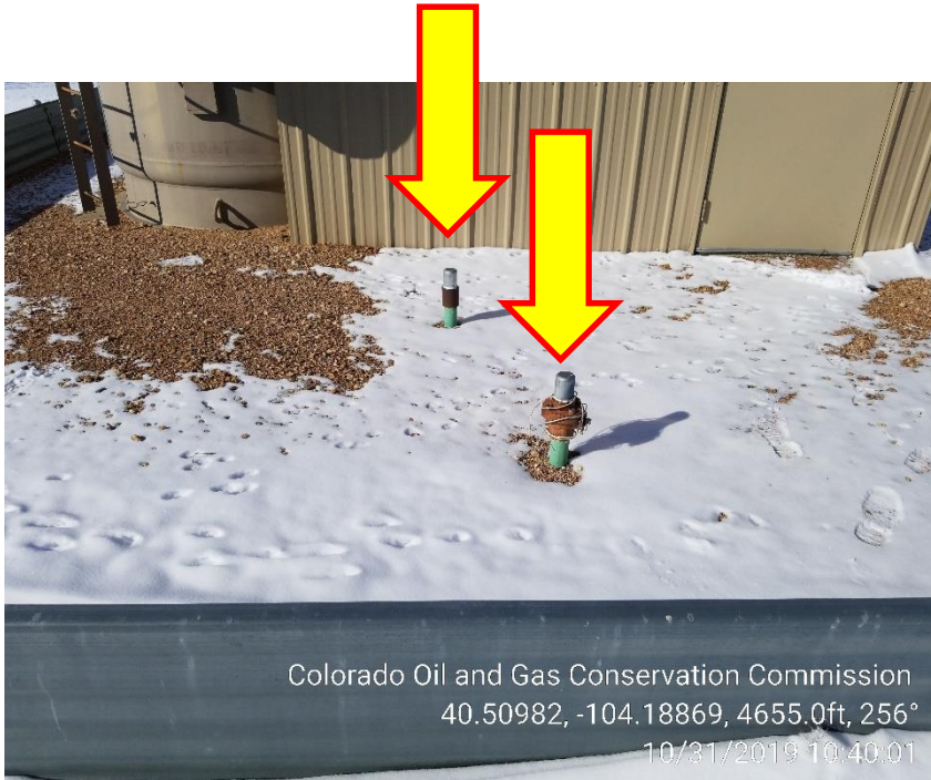
Photo 5 – Unmarked 2” Risers on the East side of the Treater House
