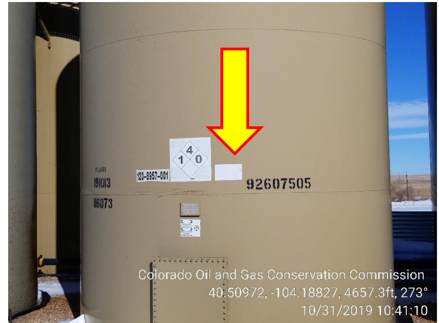
Photo 6– South Middle Tank Content and Capacity label is faded no longer legible
