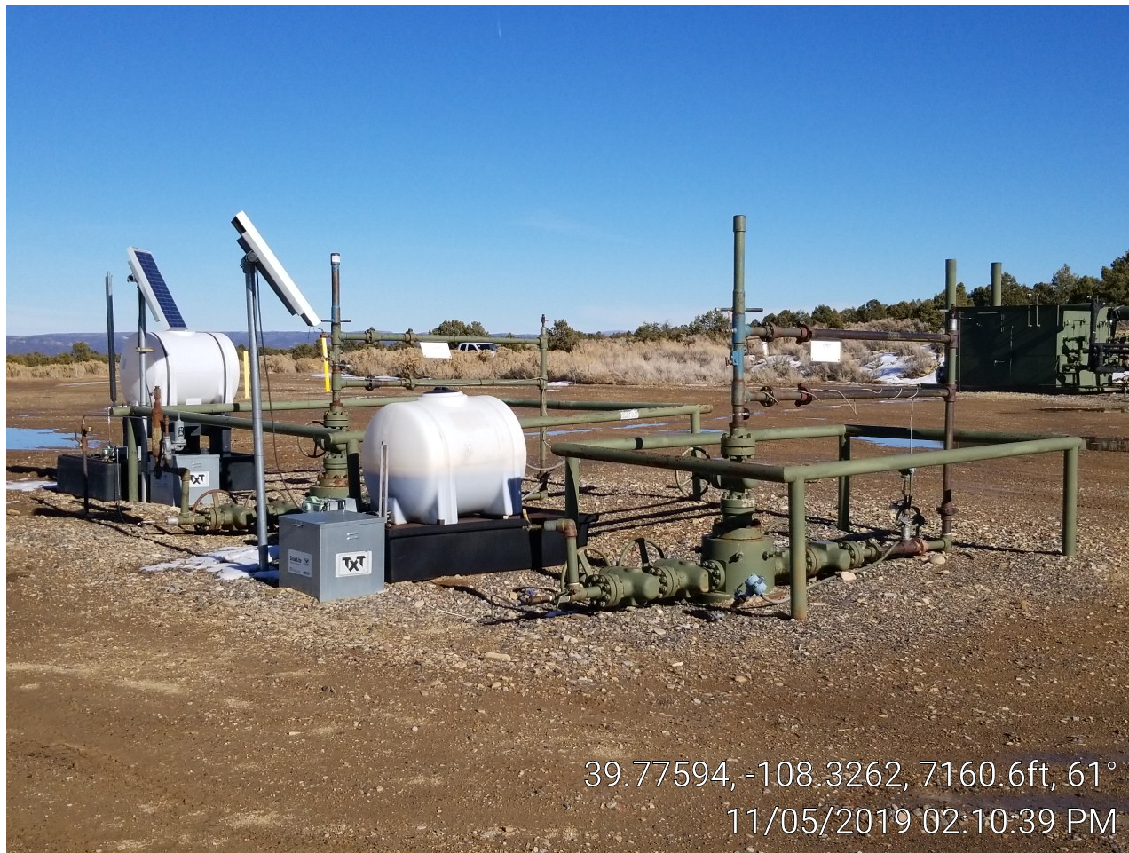
Photo 3. Well head & separator.
