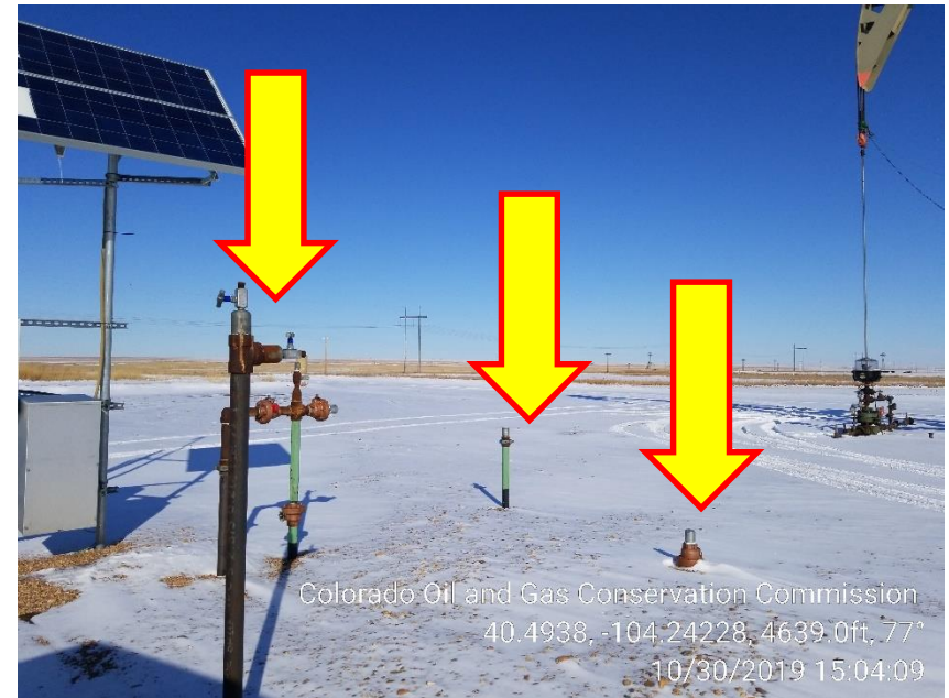
Photo 2 – Unmarked 2" Risers
