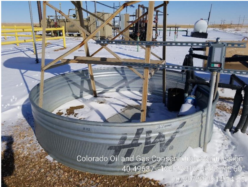
Photo 3 – Glycol Day barrel containment is missing Wildlife netting
