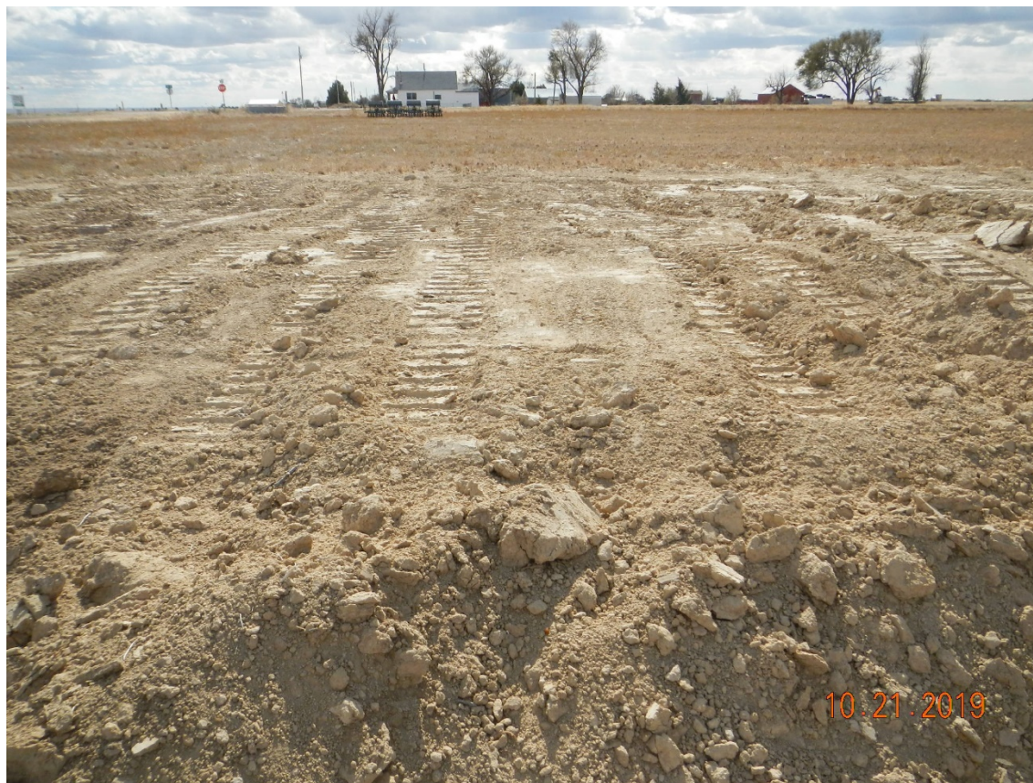
Photo # 2 – View south, pit berms pushed into pit
