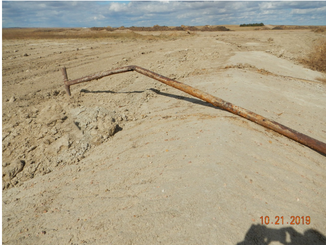
Photo # 3 – View north, siphon pipe across partial pit dividing berms requires removal, pit berm requires pH, EC and SAR analysis
