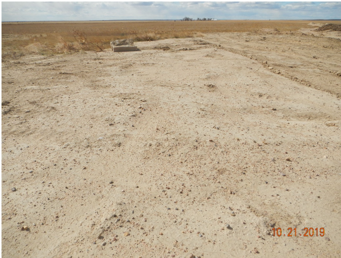
Photo # 6 – Former separator area, gravelly soil requires pH, EC and SAR analysis
