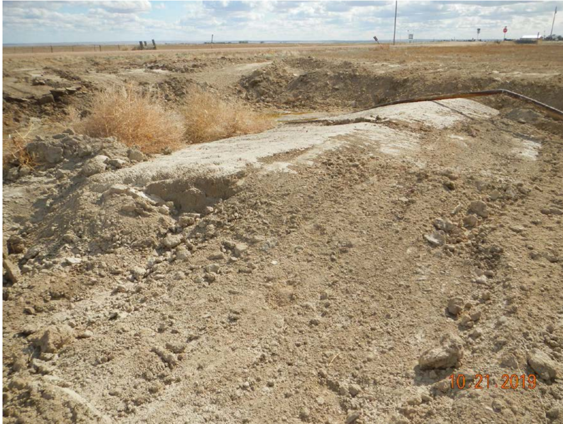
Photo # 5 – View south, siphon pipe across partial pit dividing berms requires removal, pit berm is not three feet below grade
