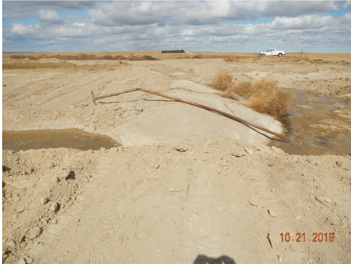
Photo # 5 – View north, siphon pipe across partial pit dividing berms requires removal
