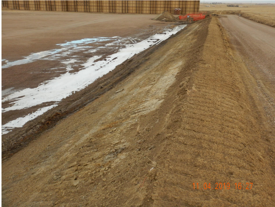
Photo 4. Photo taken from the southern location, facing East. Photo illustrates Operator has temporarily stabilized the top slope (berm) of the cut slope with hydromulch.
