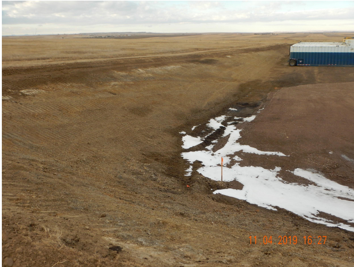
Photo 3. Photo taken from the southwestern location, facing North. Photo illustrates the cut slopes have been temporarily tracked with equipment. Note: tracking should be conducted perpendicular to the slopes. Tracking as shown here was done the opposite and would facilitate stormwater flow which would create rills that form gully erosion. Operator shall stabilize the cut slopes for long-term stabilization to comply with site degradation rule 1002.f.
