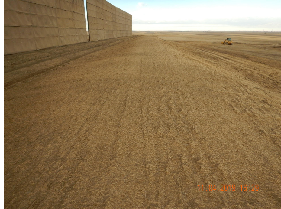
Photo 5. Photo taken from the eastern location, facing North. Photo illustrates the topsoil stockpile has been temporarily stabilized with hydromulch and equipment tracking.
