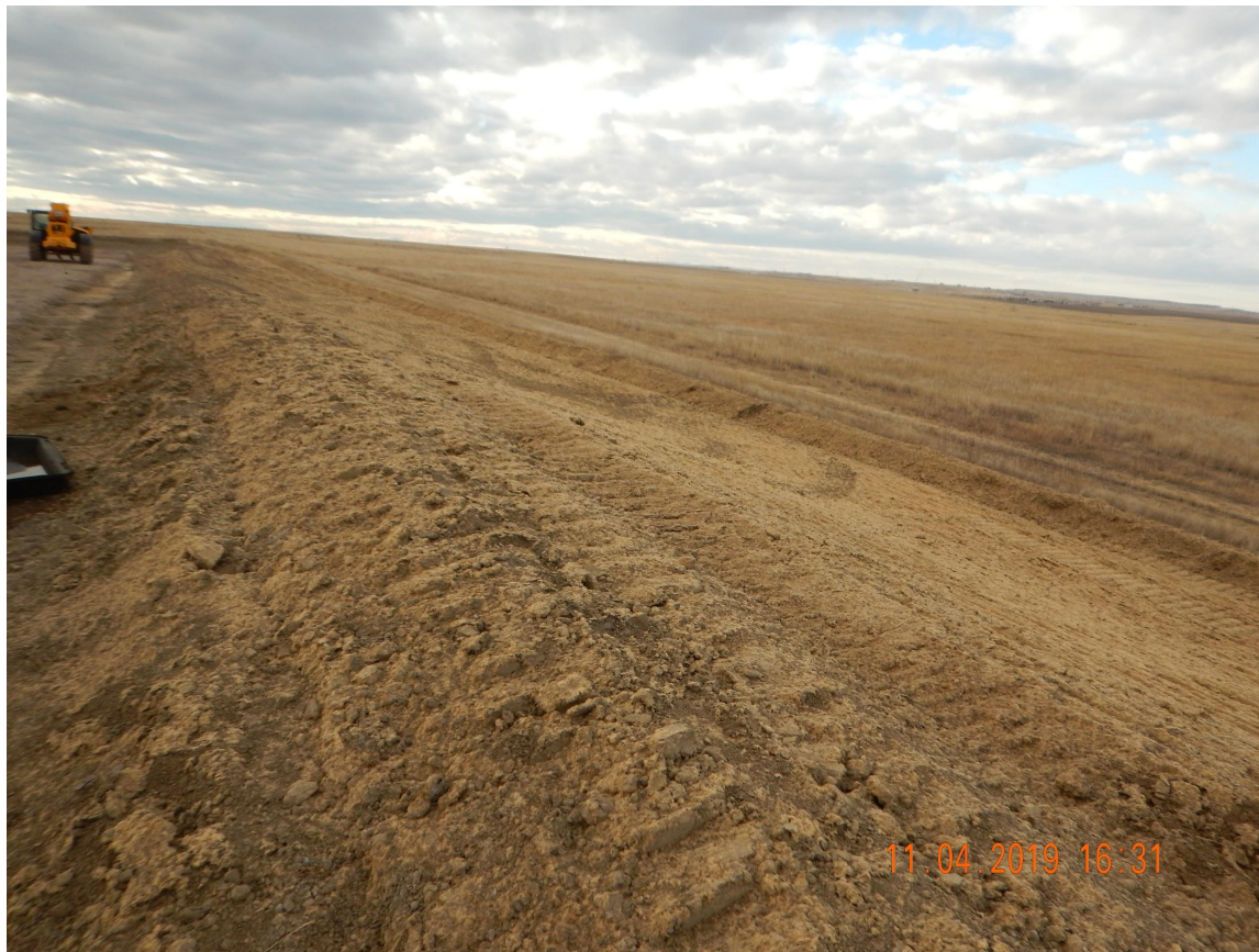
Photo 7. Photo taken from the northeastern location, facing West. Photo illustrates the fill slope has been temporarily stabilized with hydromulch.
