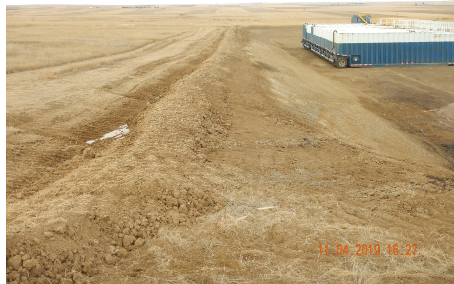
Photo 2. Photo taken from the southwestern location, facing North. Photo illustrates a ditch and berm BMP which has been temporarily stabilized with hydromulch.
