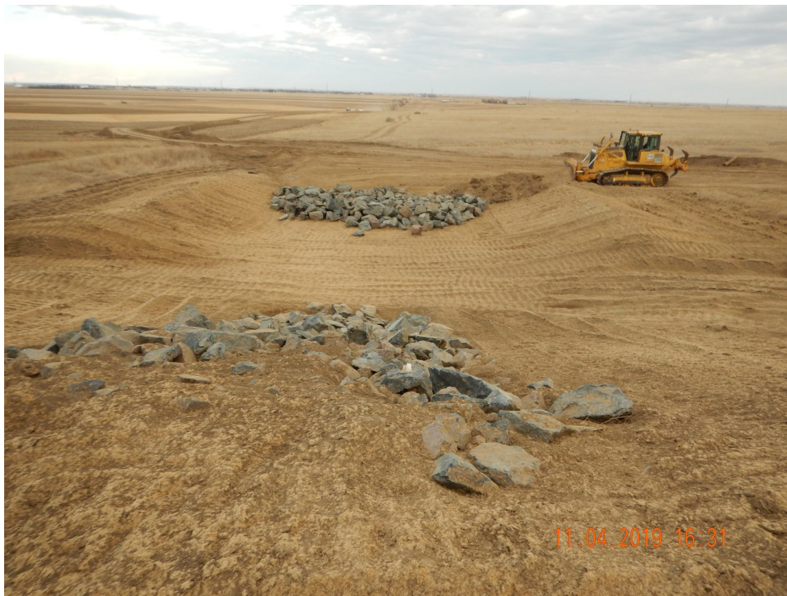
Photo 6. Photo taken from the northeastern location, facing East. Photo illustrates a sediment trap installed with a stabilized outlet. Appears the outlet material may have been compromised due to the pipeline installation.
