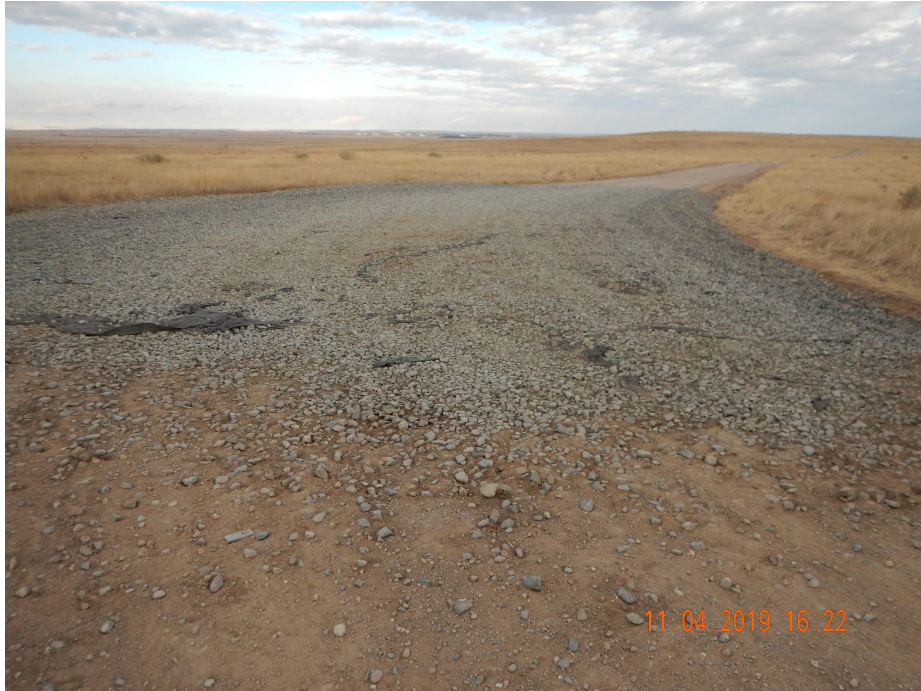
Photo 1. Photo taken from the entrance of location, facing East. Photo illustrates Operator has installed a vehicle tracking device BMP.
