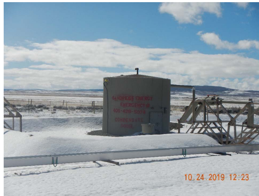
Photo 2. No NFPA diamond on tank label.
