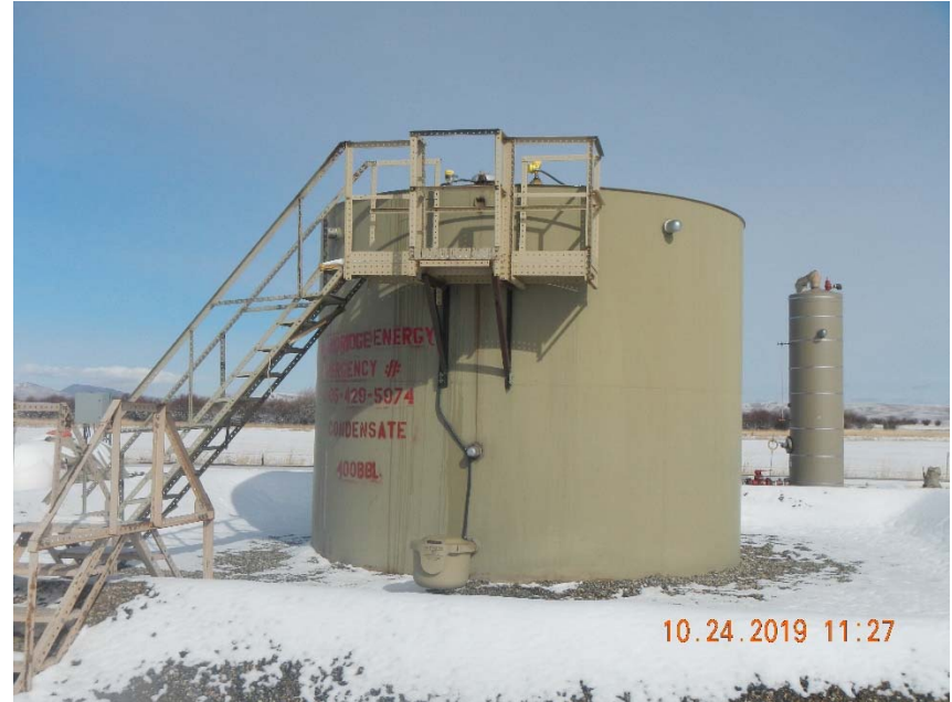
Photo 2. No NFPA diamond on tank label.
