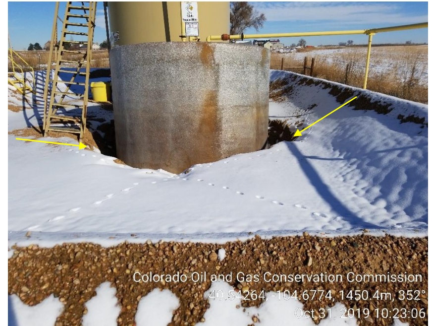
Photo 4: Sunk in base of tank battery berm
