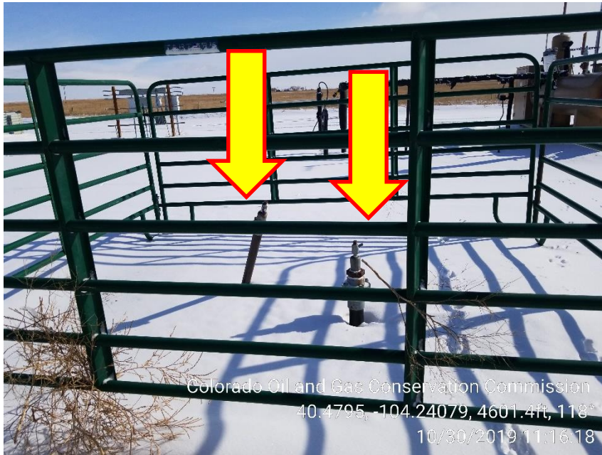
Photo 3 – Unmarked Risers
