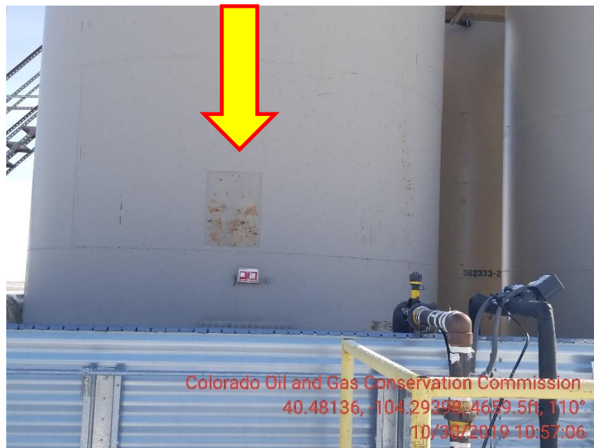
Photo 3 – NW Tank missing Content and Capacity
