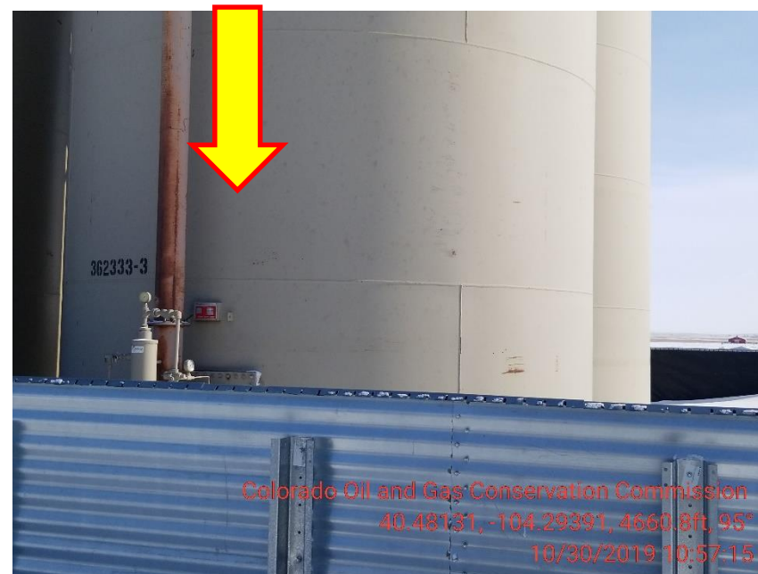
Photo 4 – SW Tank missing Content and Capacity
