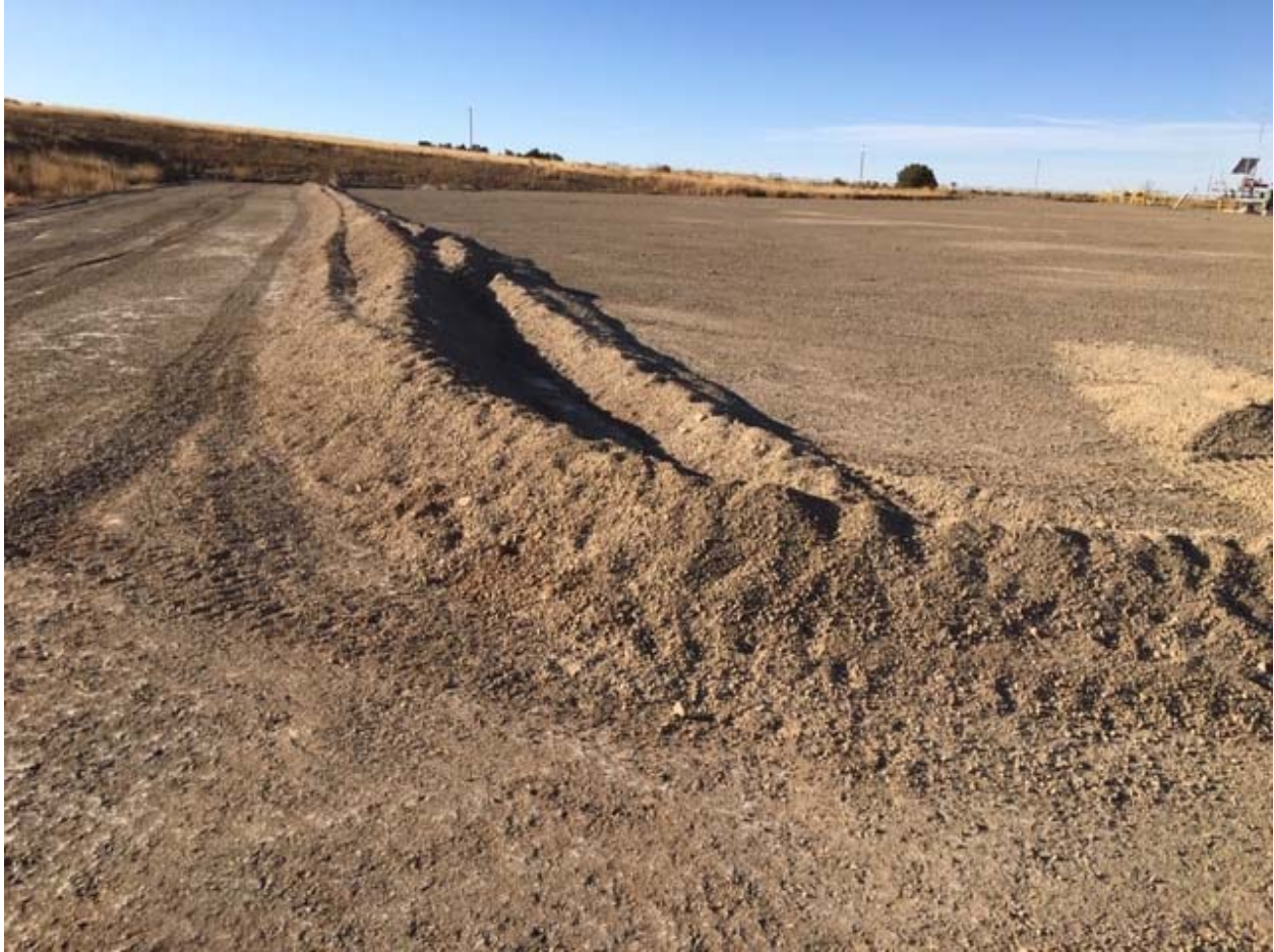
Windrowed 3/4-inch gravel on the east side of the CD-3 location
