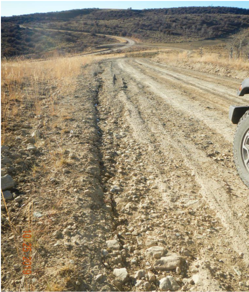
Photo#3: Ditches on either side of Access road need maintenance
