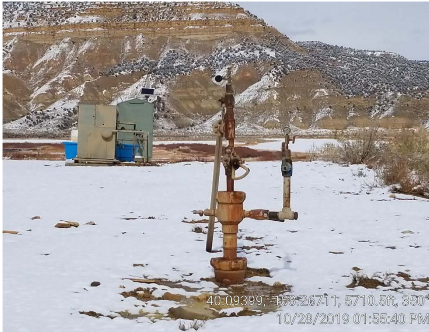
Photo 2. Well head, separator, gas meter building.
