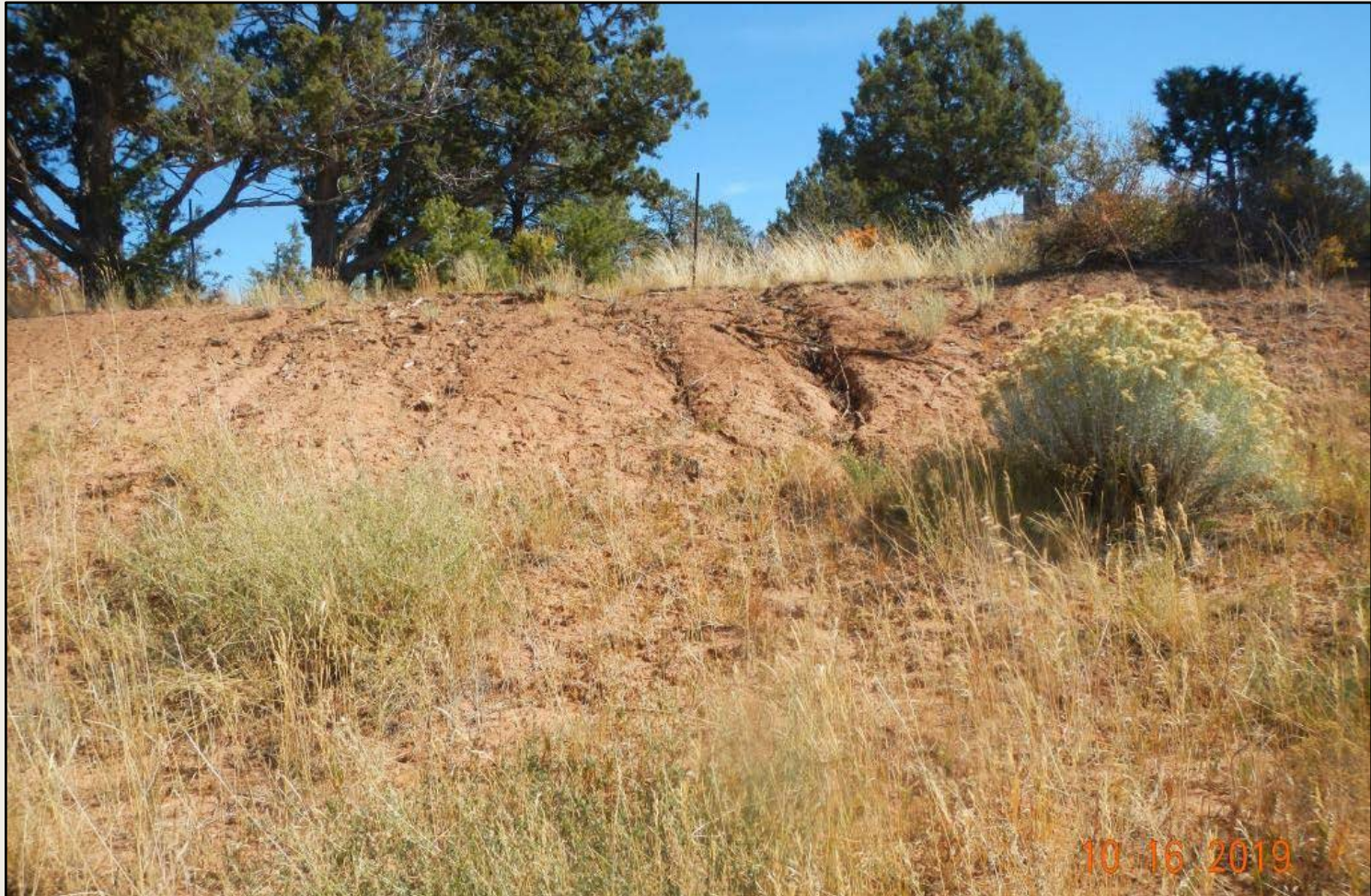
Photo 2. View of erosional channel and bare soils within the well pad cut-slope.
