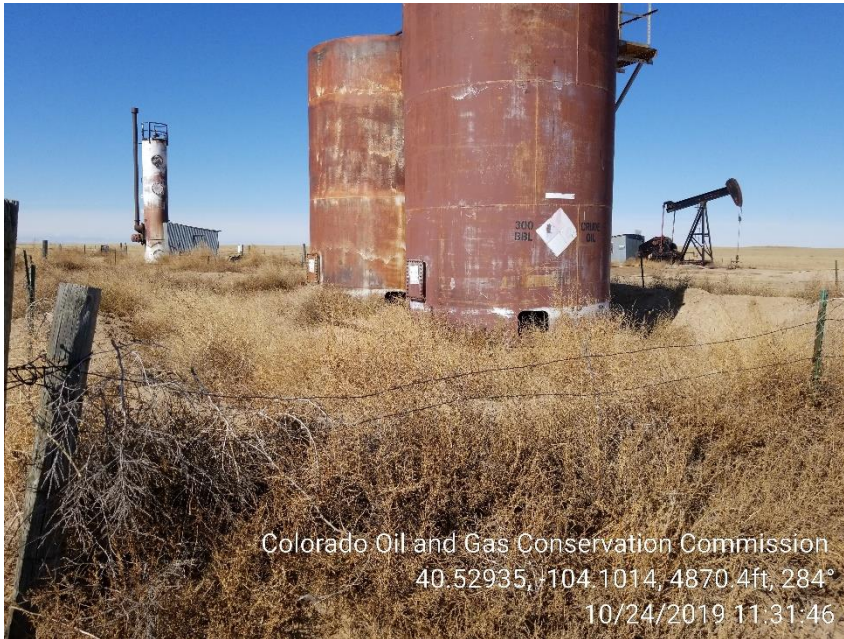
Photo 3 – Weeds at Crude Oil Tanks. Tanks are rusted, paint is peeling
