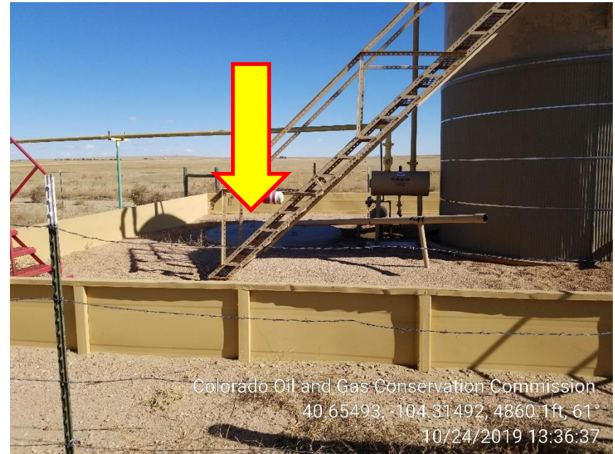
Photo 4 – PBV Concrete vault is missing Content and Capacity
