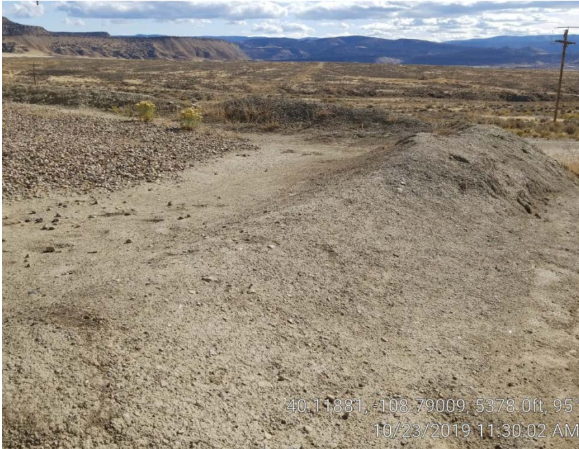
Photo 8. Berm height too short for crude oil tanks.
