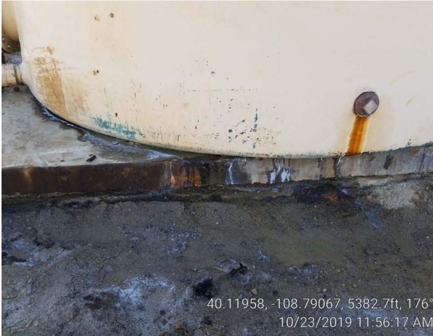
Photo 6. Water tank leak on north side.
