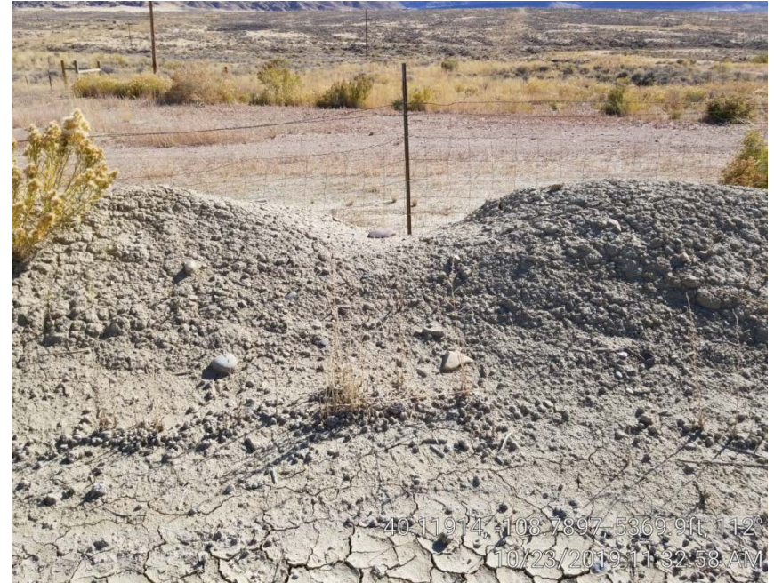
Photo 9. Berm low spot for open top tank.
