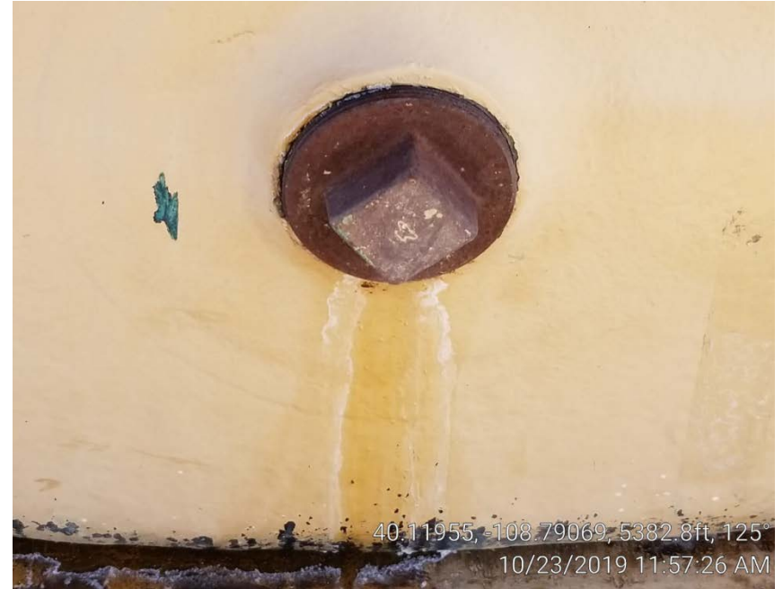
Photo 7. Water tank leak on west side.
