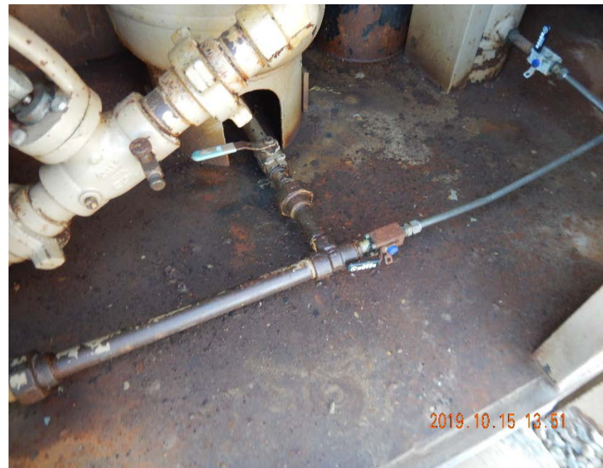
Photo #8 – Hydrocarbon odors observed in vicinity of staining on heated horizontal separators.
