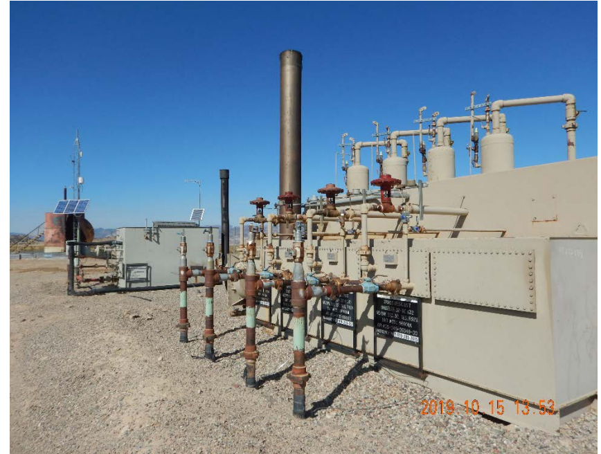
Photo #6 – View of (1) horizontal and (4) vertical separators from south.
