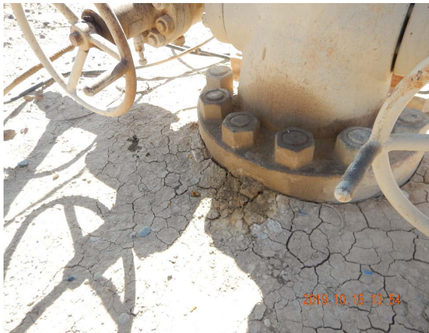
Photo #11 – Localized accumulations of oil-stained soil beneath wellhead for Graham 32-12A.
