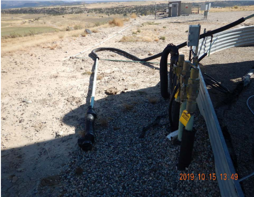
Photo #5 - Flowline risers and damaged equipment located northeast of tank (2).
