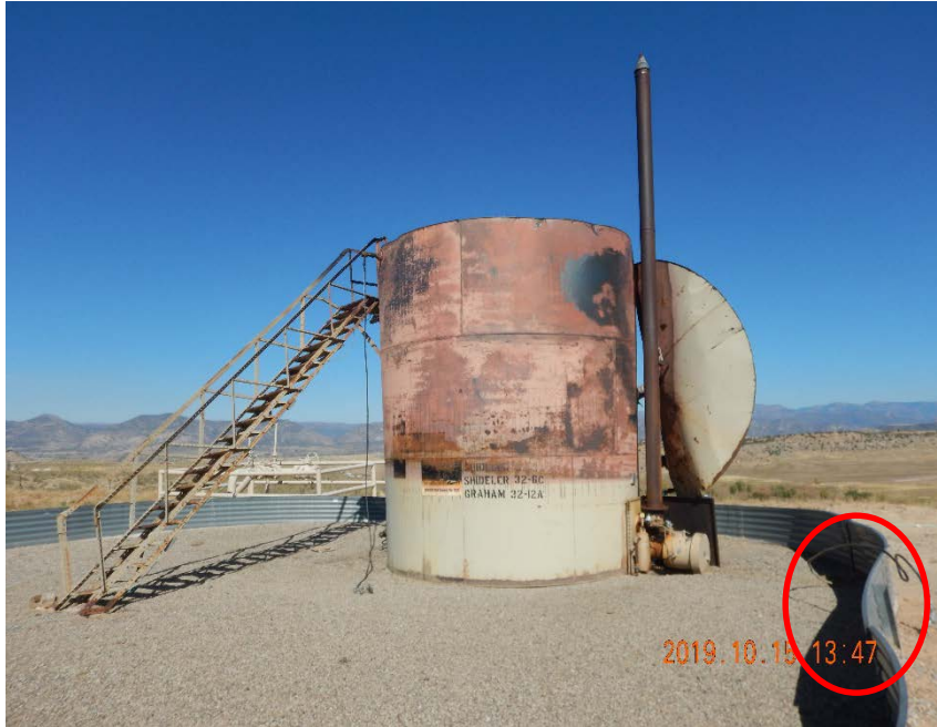
Photo #3 – View of damaged condensate AST from west. Note top blown off tank and metal berm damaged (red circle).
