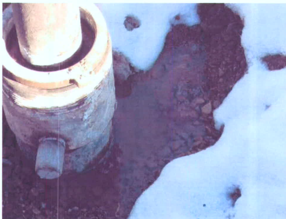
Photo 2: Methane seepage next to surface casing for Flagg #6-3 production well.
