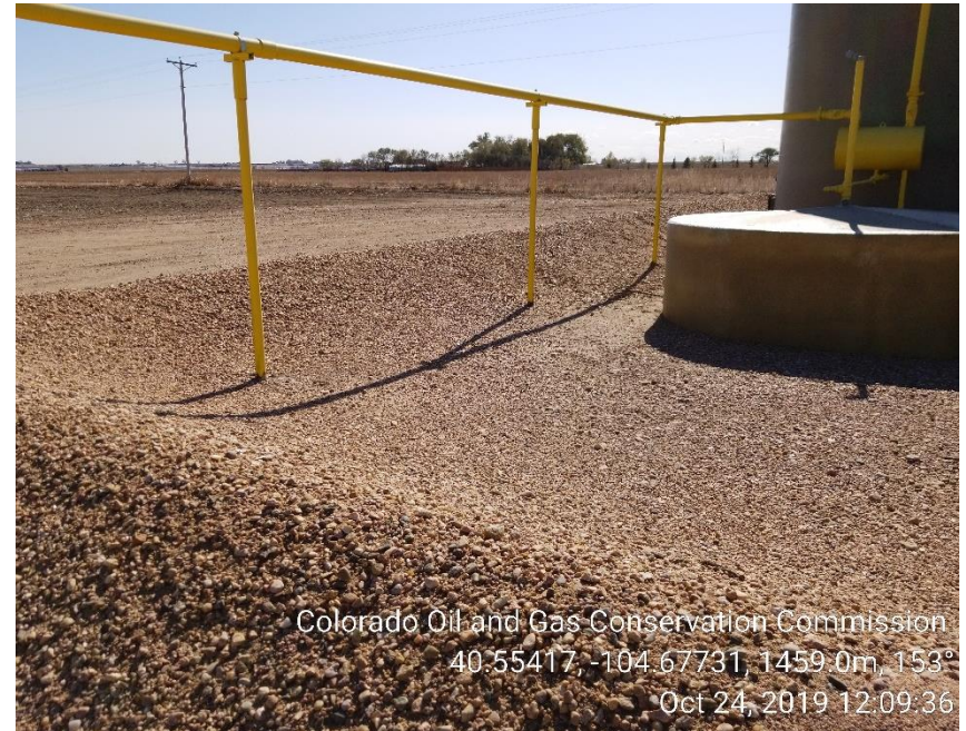
Photo 4: Berm repaired
