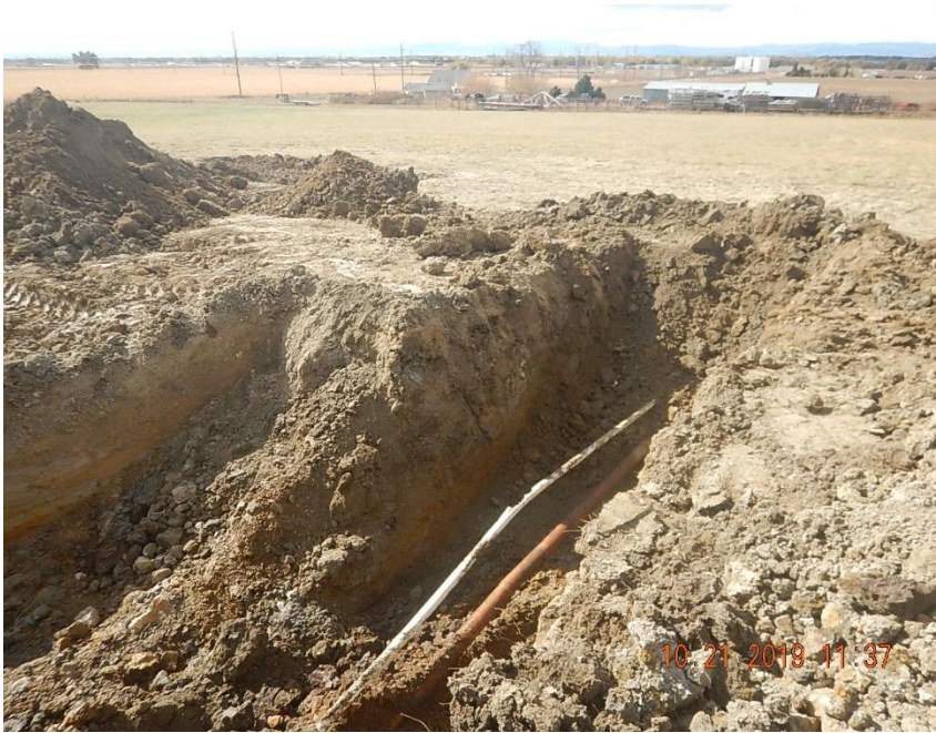
View of off location flowlines exposed in excavation (1.5" PVC gas supply line & 3" fiberglass wellhead flowline); looking SW
