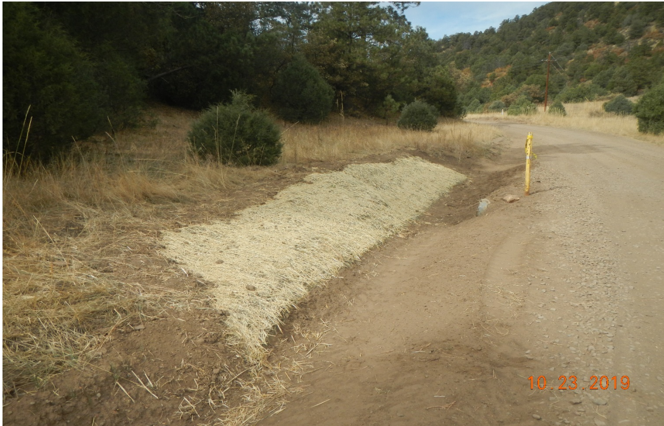
Photo 1. The culvert has been cleaned out of sediment. Straw blanket was installed in the disturbance area.
