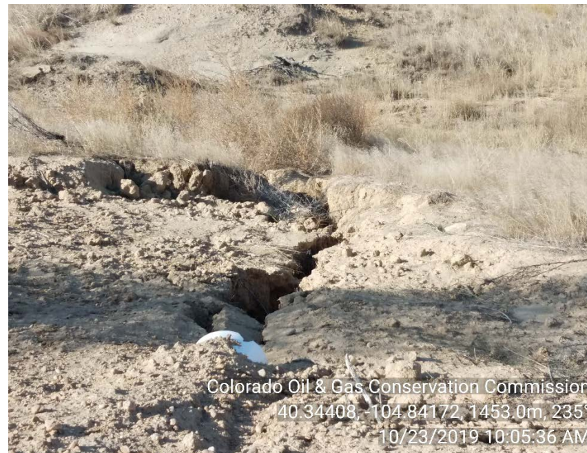
PVC pipe culvert and off site erosion
