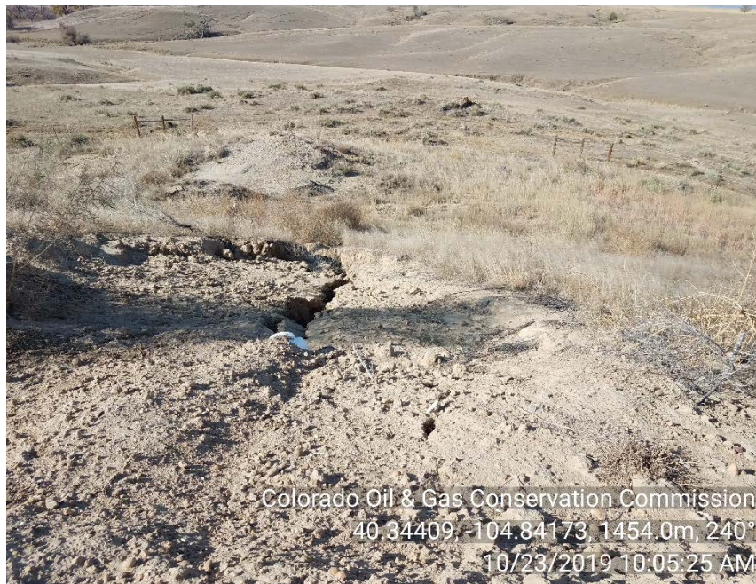
PVC pipe culvert and off site erosion
