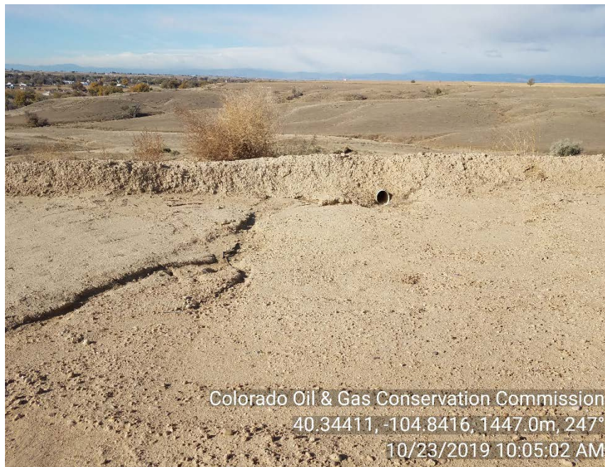
West berm wall and PVC pipe culvert
