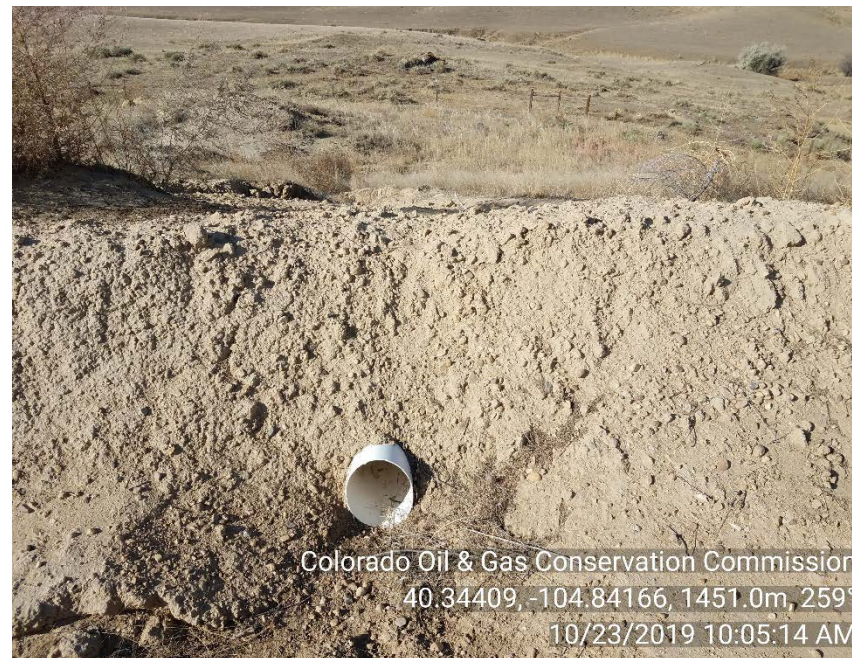
West berm wall and PVC pipe culvert
