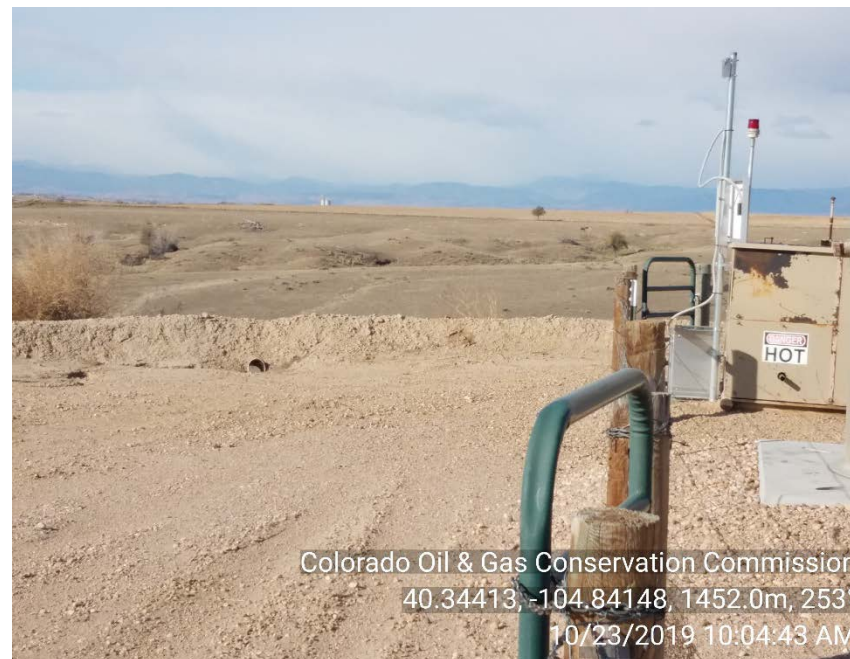
West berm wall and PVC pipe culvert
