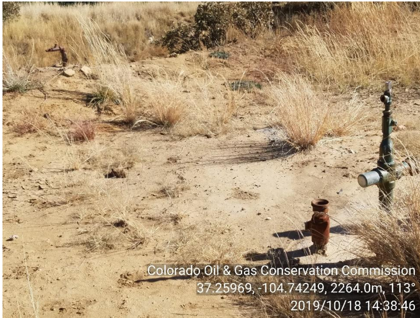
PHOTO 3: 3 UNMARKED UNUSED RISERS, ONE 1" AND TWO 2" RISERS NEAR ORIGINAL WELLHEAD. REMOVE RISER COMPLY WITH NTO. CA DATE 11-18-19
