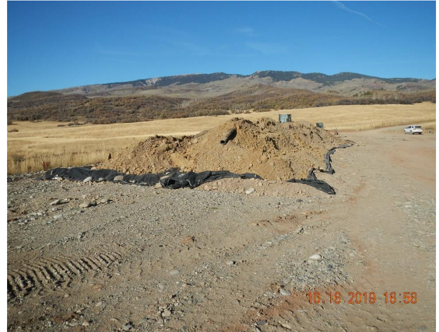
Insufficient containment for impacted material.
