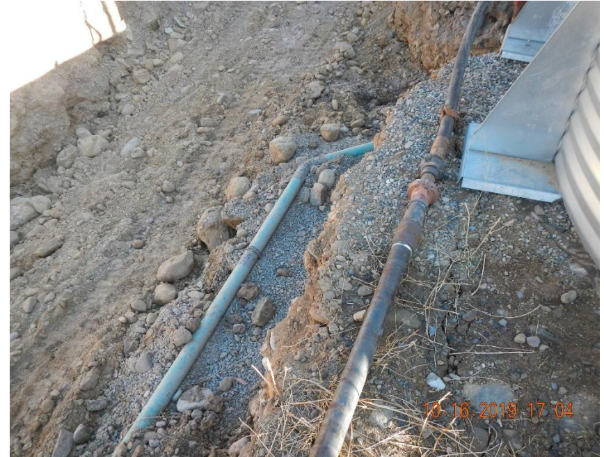
Replacement above ground dump line.
