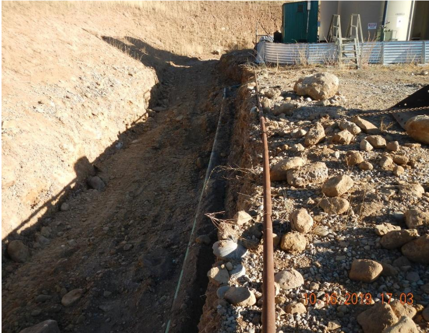
Above ground replacement dump line anchored by chains to skid steer and secondary containment stairway railing.
