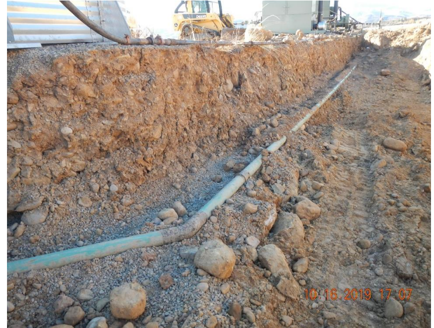
Excavated dump line from separators to tank battery.
