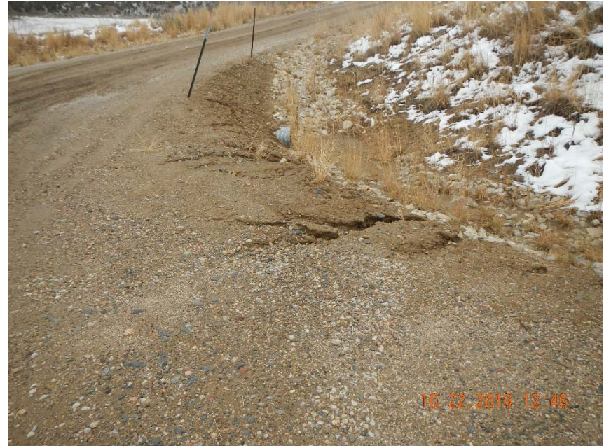
Photo 5. Rills and sediment leaving location.
