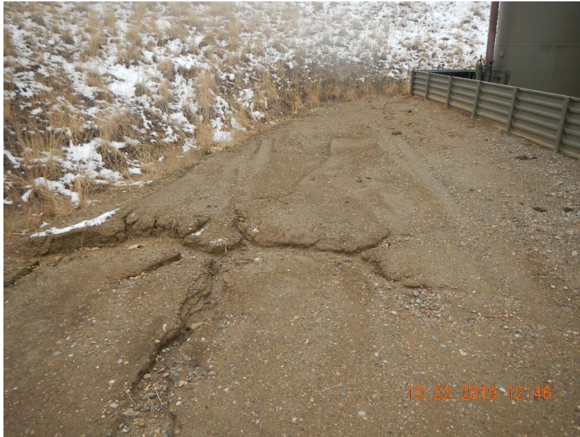
Photo 4. Rills and sediment leaving location.
