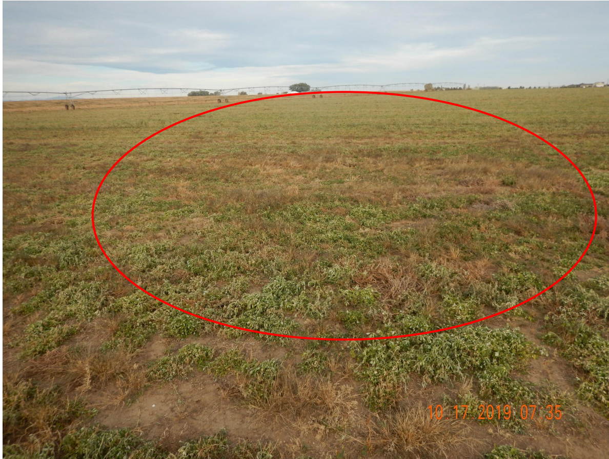
Photo 1. Photo taken from the well location, facing North. Photo illustrates the well location has not been properly re-contoured to match the surrounding landscape and/or potential subsidence occurred.
