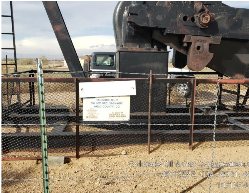
Photo #1 WH sign Operator and emergency number faded and not legible
