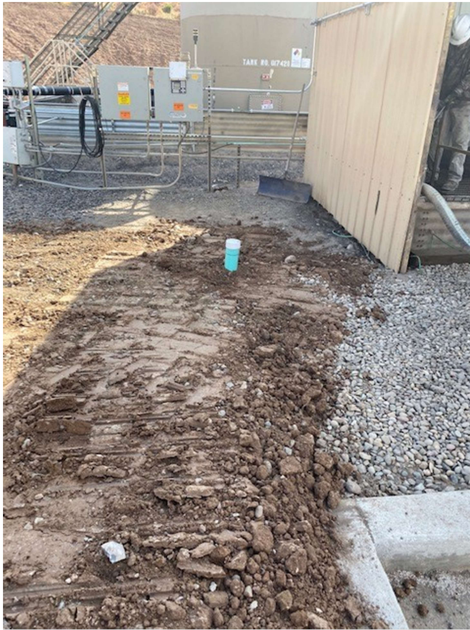
Photo 1 – Vent Installed at E1 Sample Location
